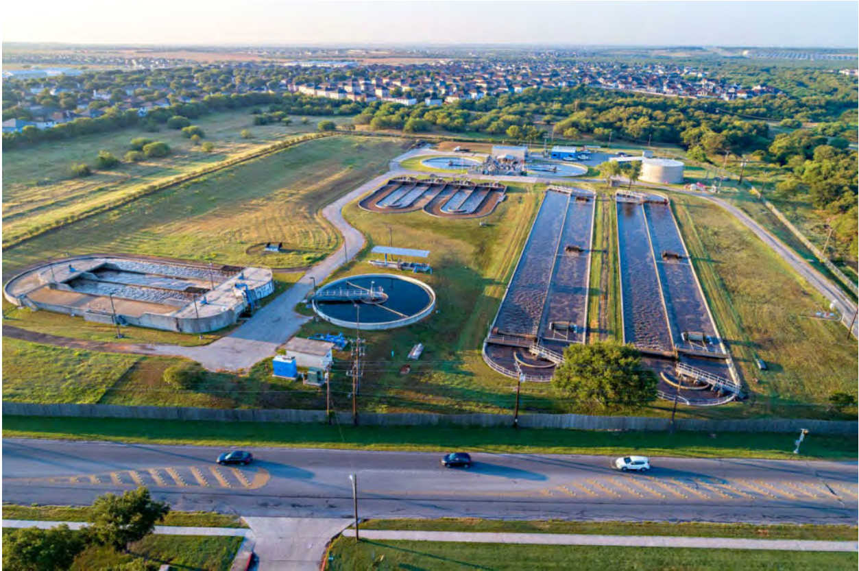
Salitrillo Wastewater Plant
