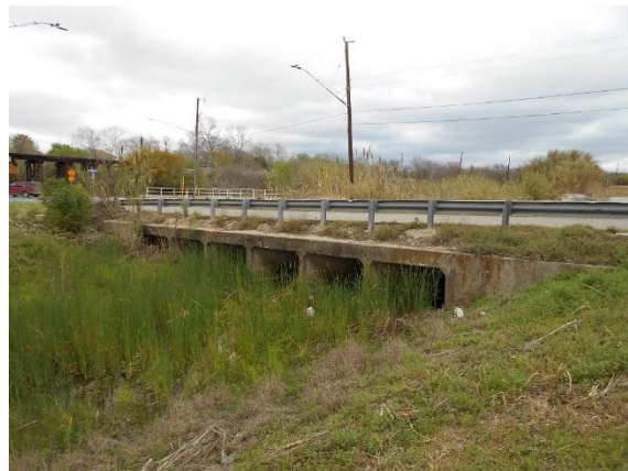
Downstream Structure Face
