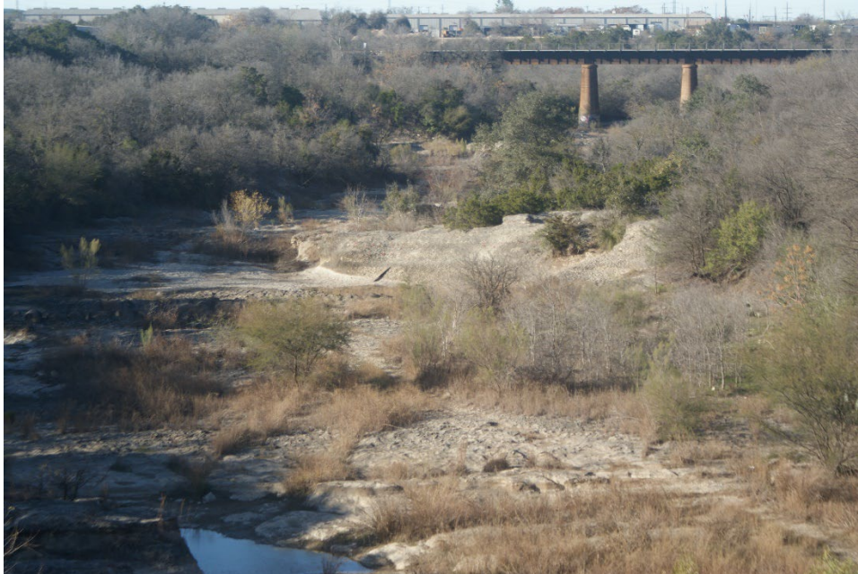
Figure 3-2: Mid Cibolo Creek upstream of Nacogdoches Road West of Bracken. Pooled water can be seen at the bottom of the picture, upstream is dry. Note the railroad bridge in the distance is the segment divider between the Upper and Mid Cibolo Creek.
