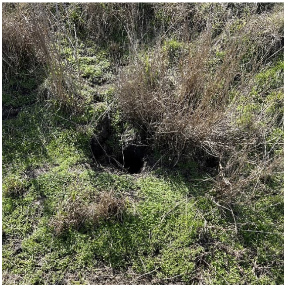
Downstream embankment showing burrows
