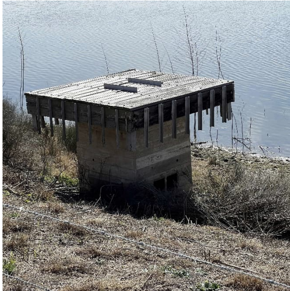
Inlet structure looking southeast with two low level ports visible
