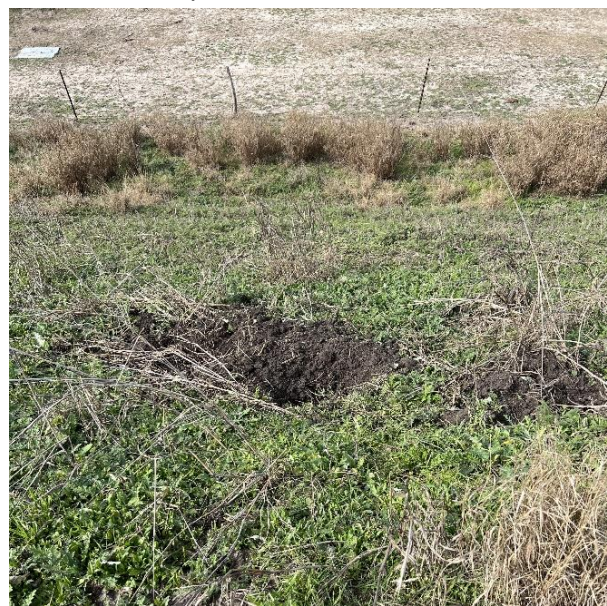
Downstream embankment showing burrows
