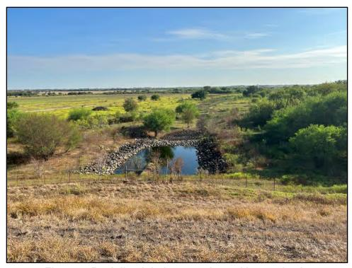
Figure 7. Rock-lined drainage outlet and impact basin
