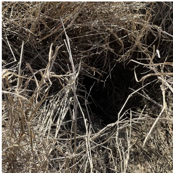
Downstream embankment showing burrows
