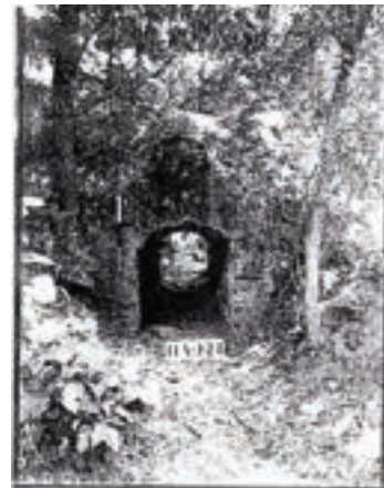
Stone bridge in 1936
