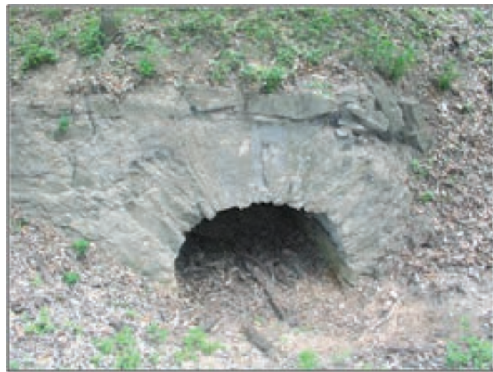
Figure 3. East face of archway.
