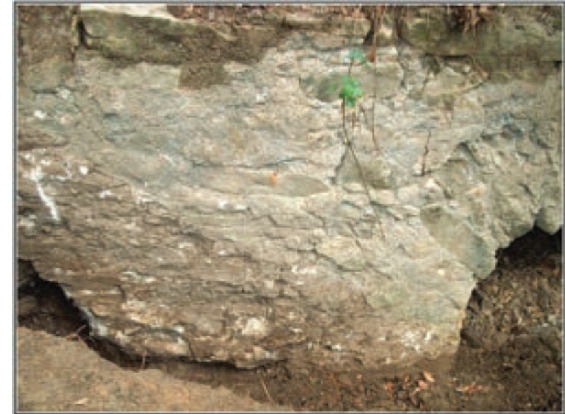
Figure 13. Base of the retaining wall along the north face of the arch.
