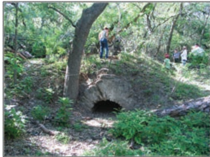
Figure 4. West face of archway.
