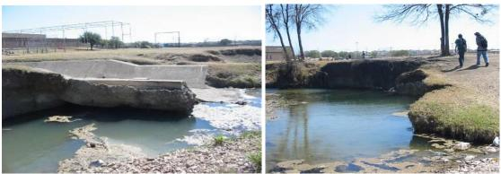
Highly eroded section adjacent to drainage Structure (Pre-Project)
