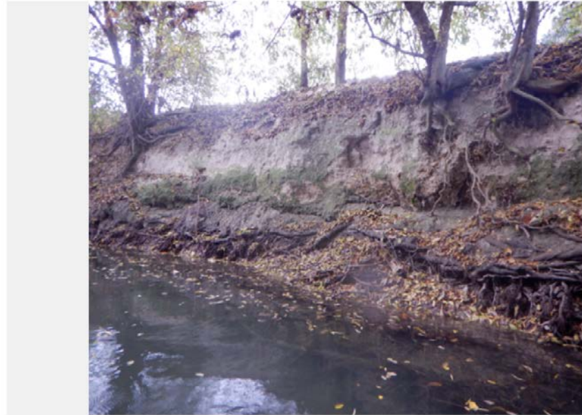
River Road Restoration Project
