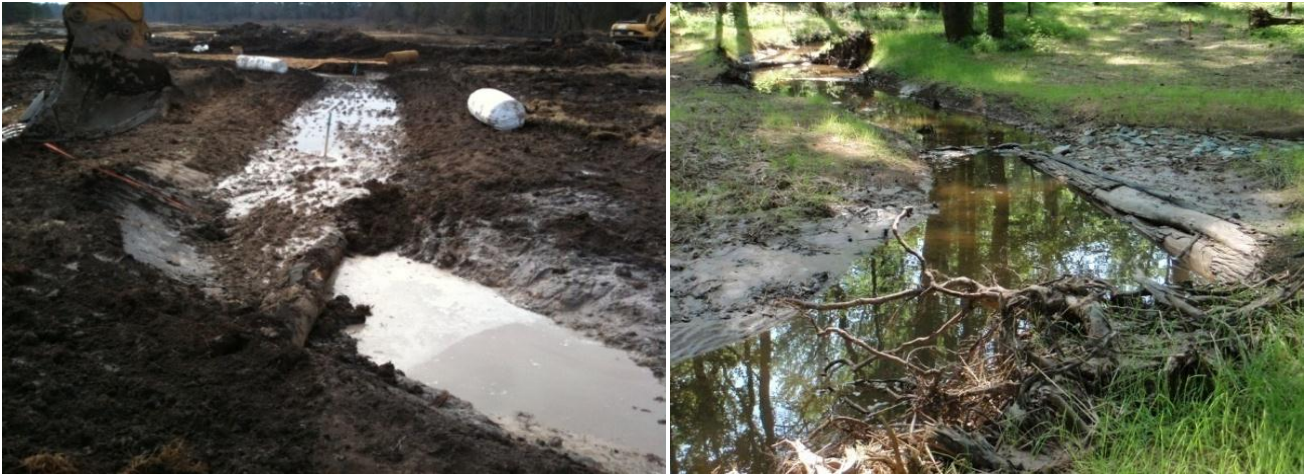
Installation of log vane during construction.
