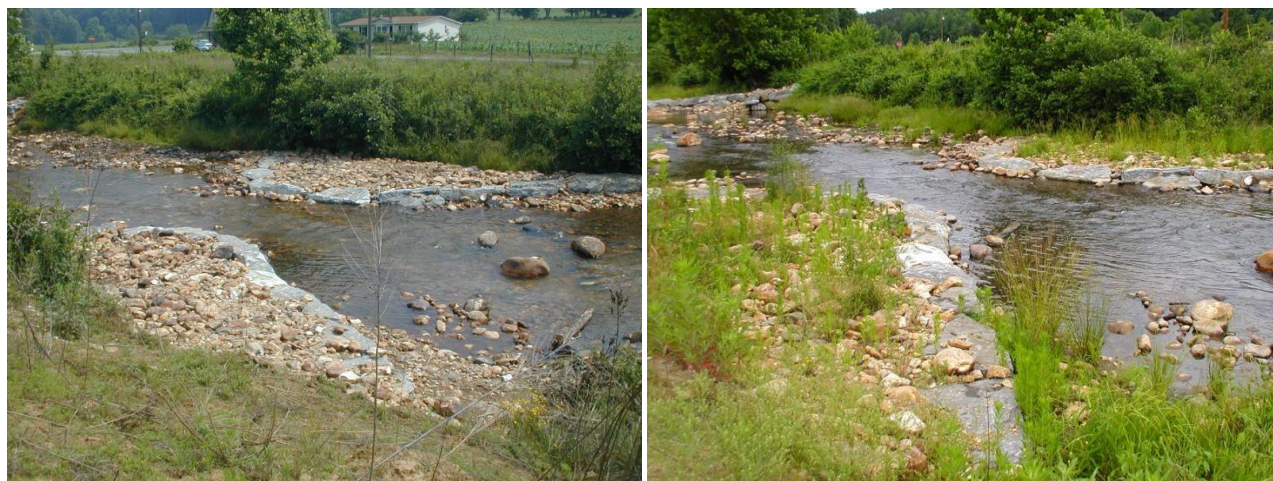
Example of double wing deflectors
