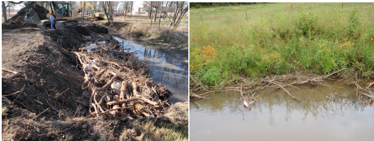
Installation of toe wood, during construction.
