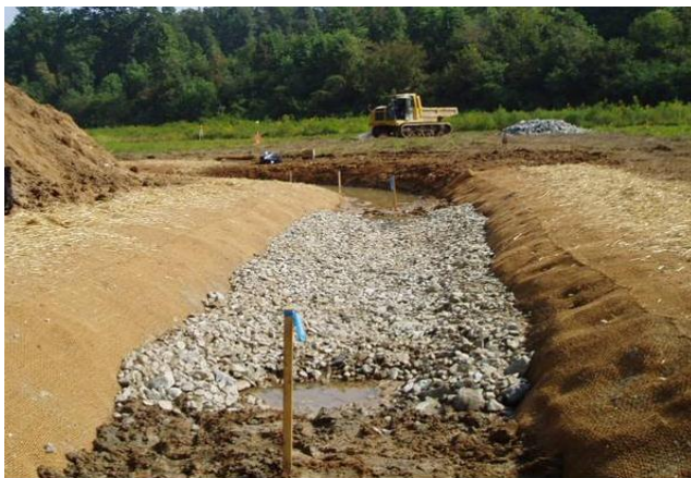
Constructed riffle during construction
