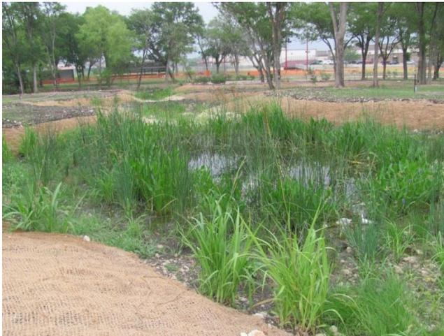
Based on site conditions and cost restrictions, the traditional bioswale design was slightly modified. Soil amendments were not included, and instead several storage areas with littoral shelves, separated by cascade riffles were designed. The cross-section for the riffle areas was sized based on the results from the Hydraulic Design tool within HEC-RAS. The littoral shelves were planted with wetland species to further aid with treatment and nutrient uptake.
