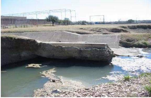
Highly eroded section adjacent to drainage Structure (Pre-Project)
