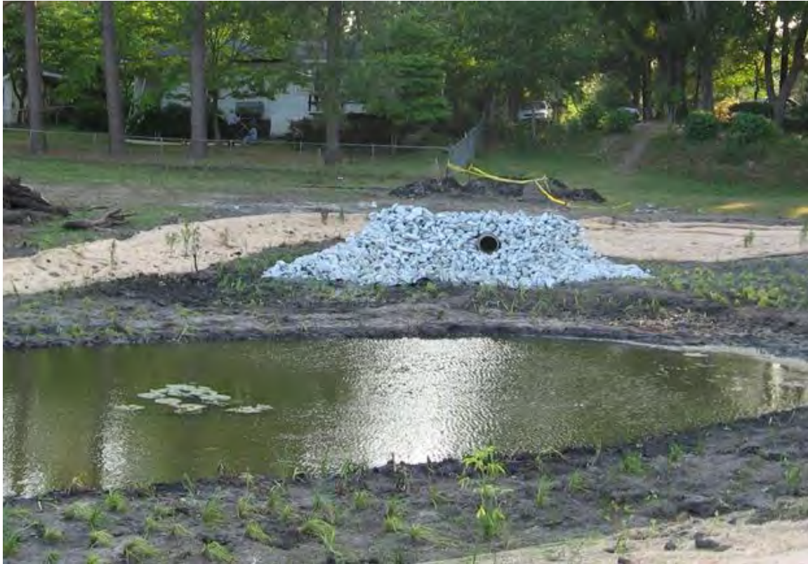
Figure B-7-2. Rock-lined forebay visible in a newly planted stormwater wetland, Wilmington, North Carolina. Source: Tetra Tech
