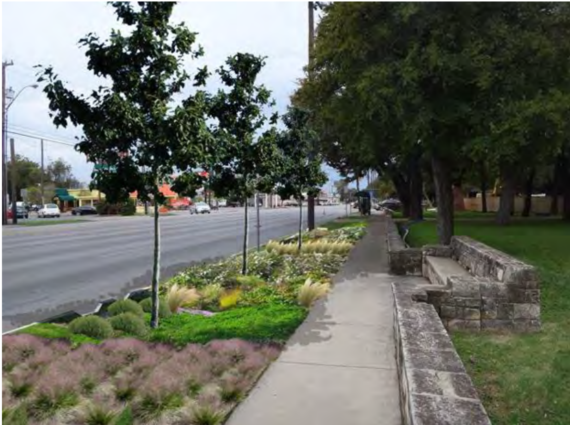
Figure 3-5. Rendering showing how roadside bioretention can be retrofit into the right-of-way to intercept street runoff through curb cuts, Broadway Street, Witte Museum, San Antonio, Texas. Source: Bender Wells Clark Design
