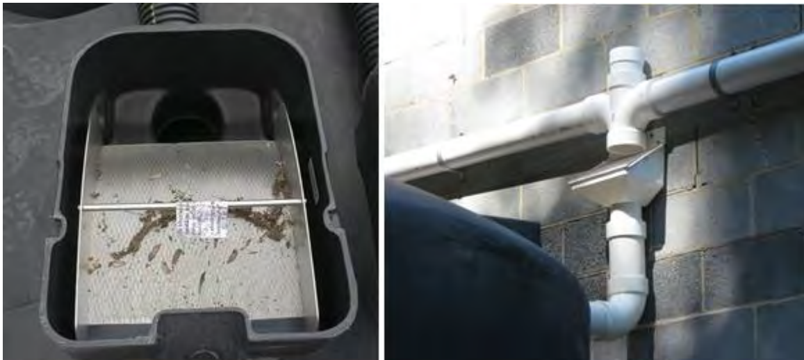
Figure 4-10. Self-cleaning inlet filters. Source: Tetra Tech
