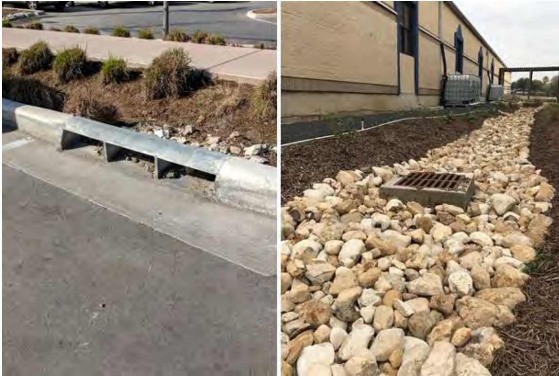
Figure B-2-6. An offline bioswale (left) along the road right of way with excess flow bypass along the gutter line at the Doseum, San Antonio Texas; and an online bioswale (right) with an overflow outlet structure along a roadway and parking lot that is part of a treatment train with an adjacent detention basin, San Antonio, Texas.
