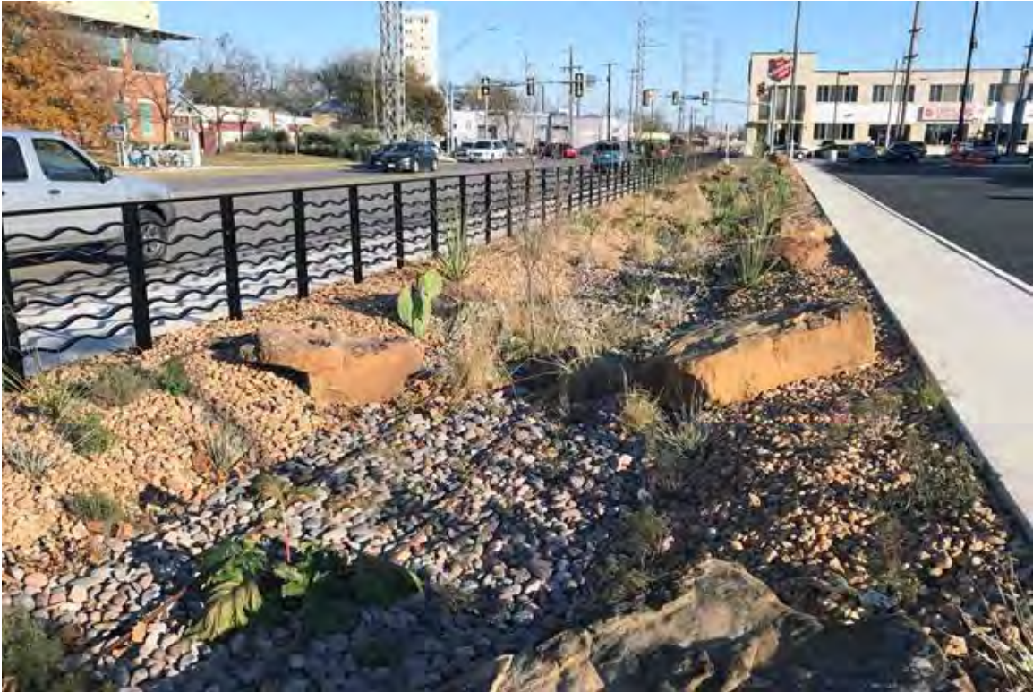
Bioswale at City of San Antonio Development Services Department parking lot, San Antonio, Texas.
