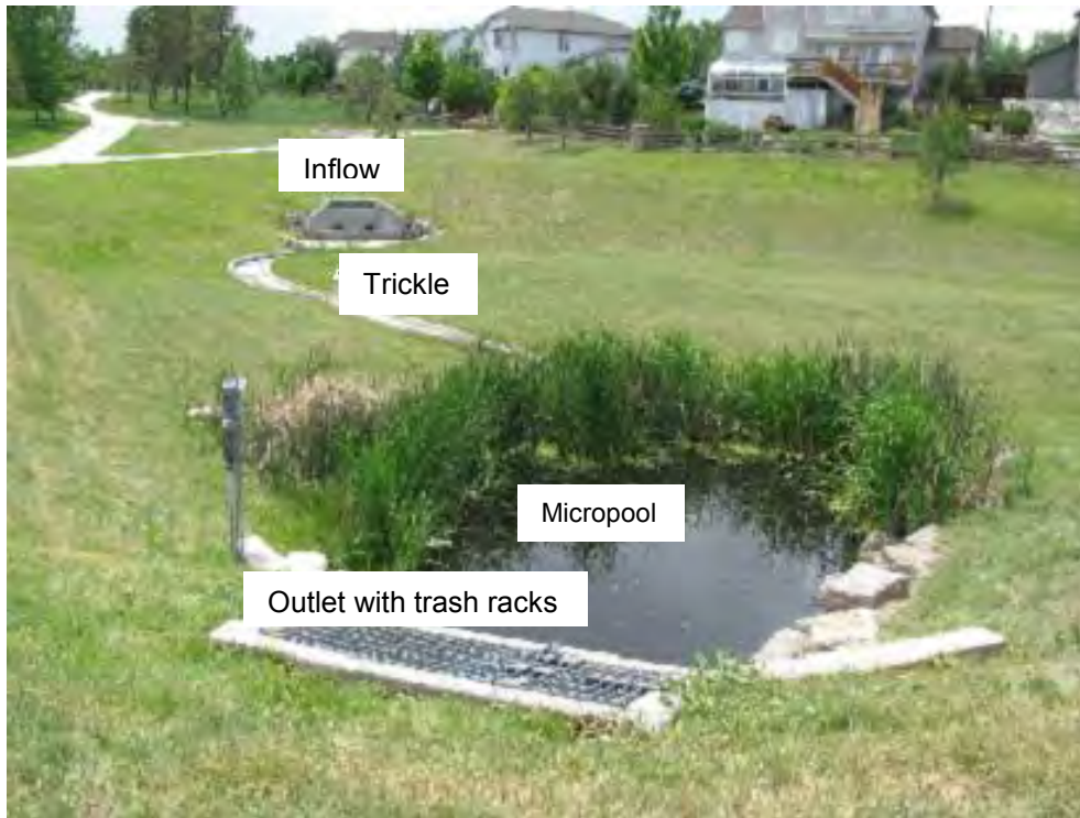
Figure 3-27. Extended Detention Basin, Grant Ranch, Colorado. Source: Urban Drainage Flood Control District
