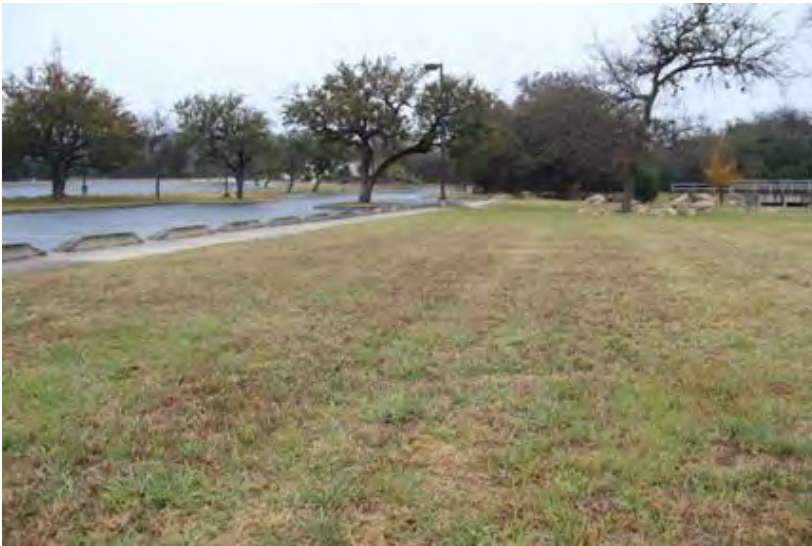
Figure 3-33. Vegetated filter strip next to a parking lot, San Antonio, Texas. Source: Tetra Tech
