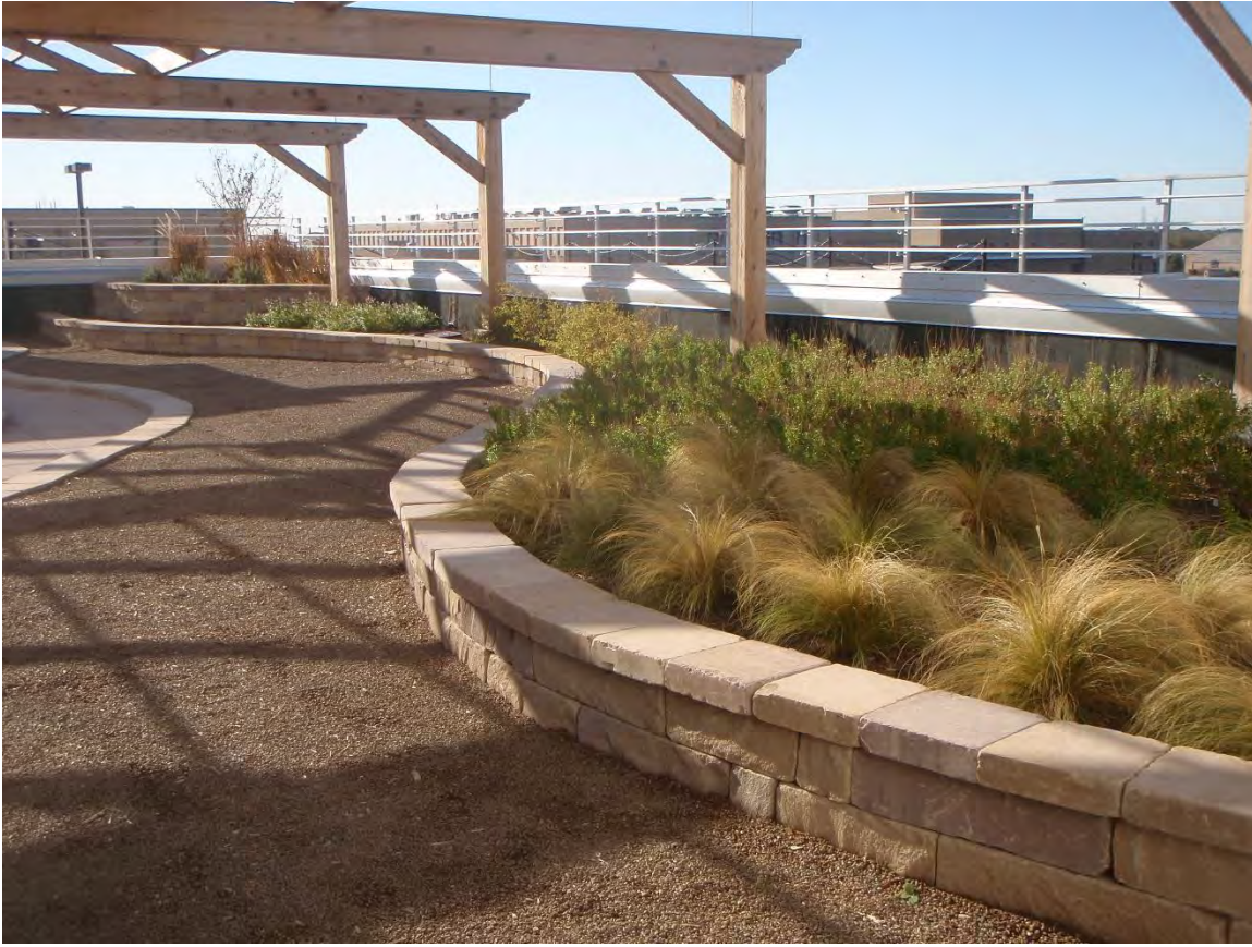
Figure B-5-2. Example of an intensive green roof at James Madison High School Agriscience Building, San Antonio, Texas. Source: Bender Wells Clark Design
