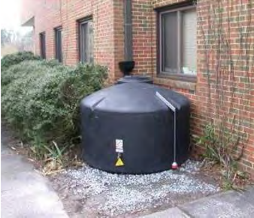
Figure B-9-2. Cistern less than 2,000 psi on a gravel foundation, New Bern, North Carolina. Source: North Carolina State University Department of Biological and Agricultural Engineering
