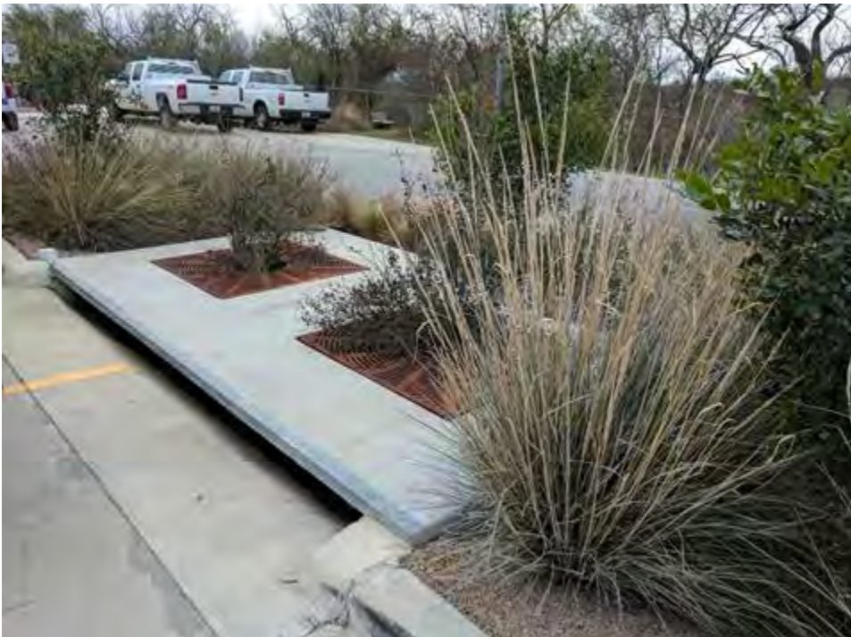
Figure 3-4. Bioretention system incorporated into parking lot, Mission Reach Operations Center, San Antonio, Texas.
