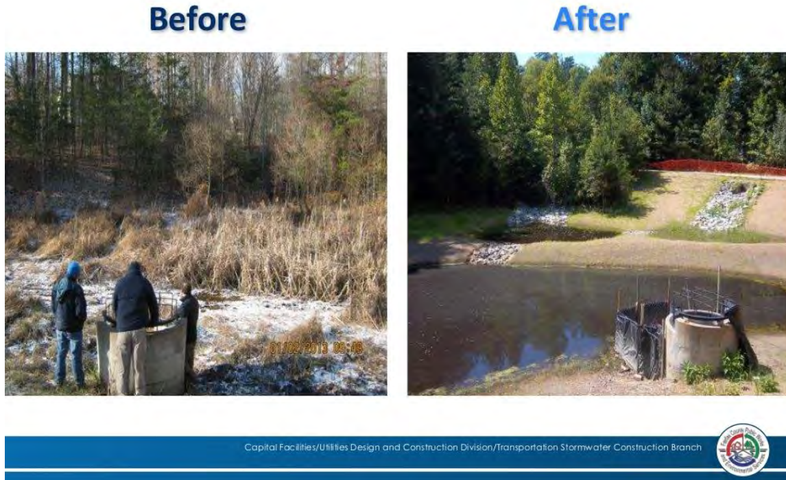
Figure 3-28. Pond retrofit before and after. Source: Crosspointe and Fairfax County, VA
