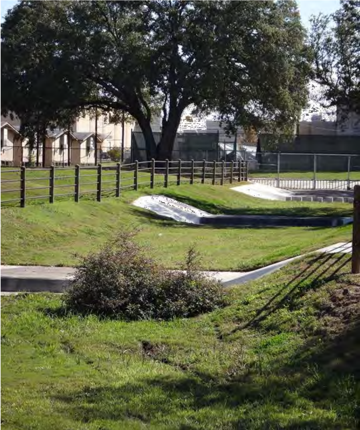
Vegetated swale at Madison High School Agriscience Building, San Antonio, Texas. Source: Bender Wells Clark Design
