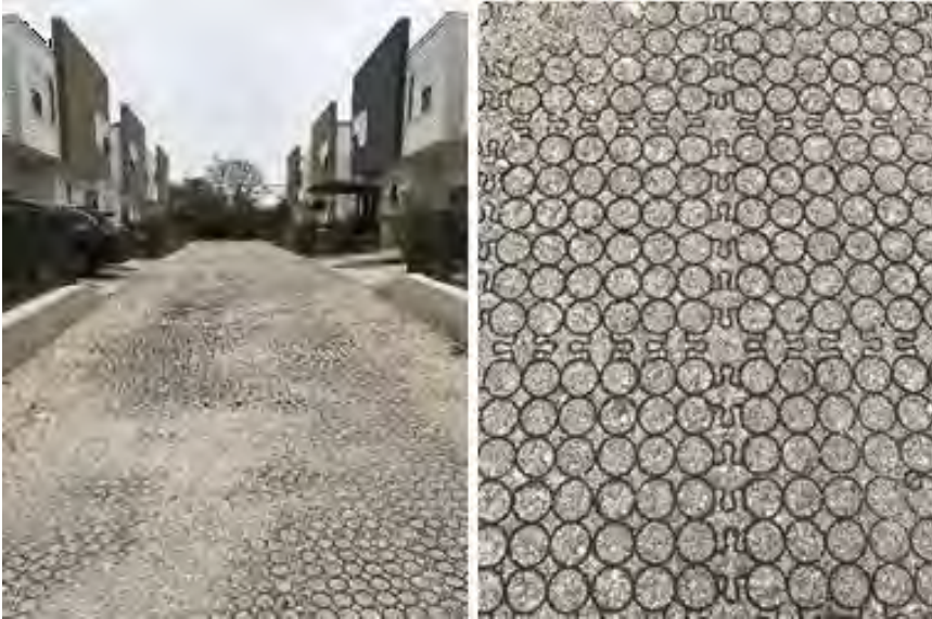
Figure B-3-10. Example of plastic grid system filled with rock that serves as a roadway for residential units, San Antonio, Texas.
