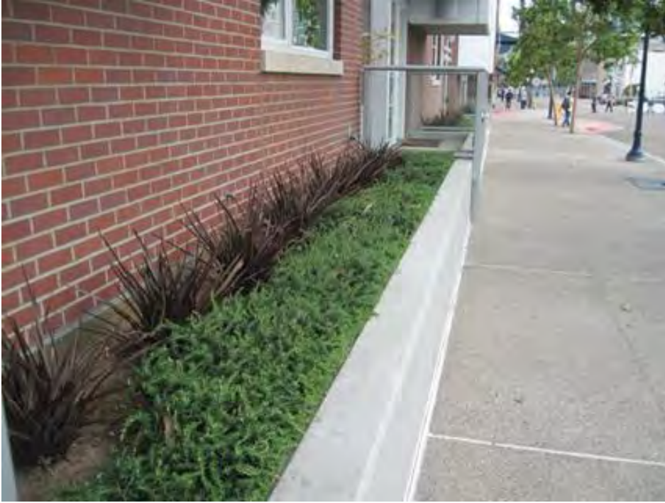
Figure 3-13. Planter boxes along a building, San Diego, California. Source: Tetra Tech
