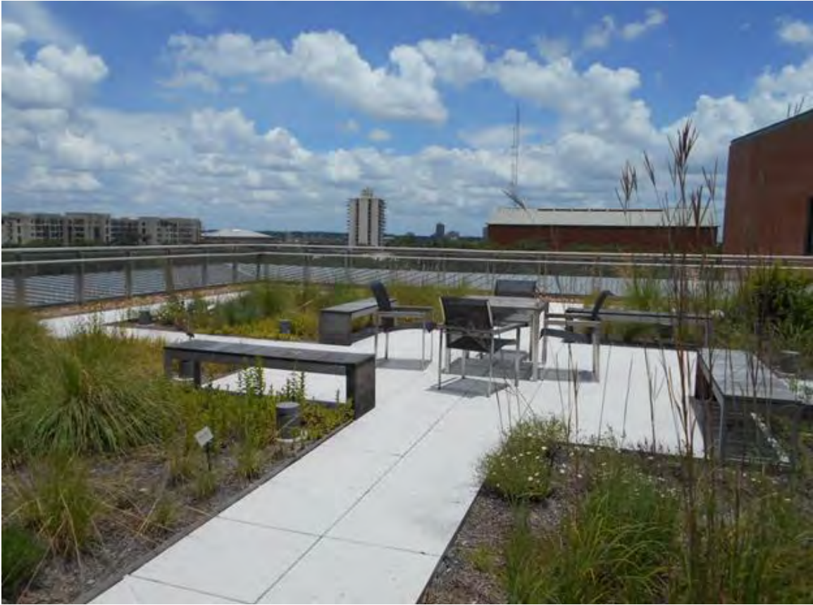
Intensive green roof that serves as a patio space at the Center for Science and Innovation. Trinity University, San Antonio, Texas.
