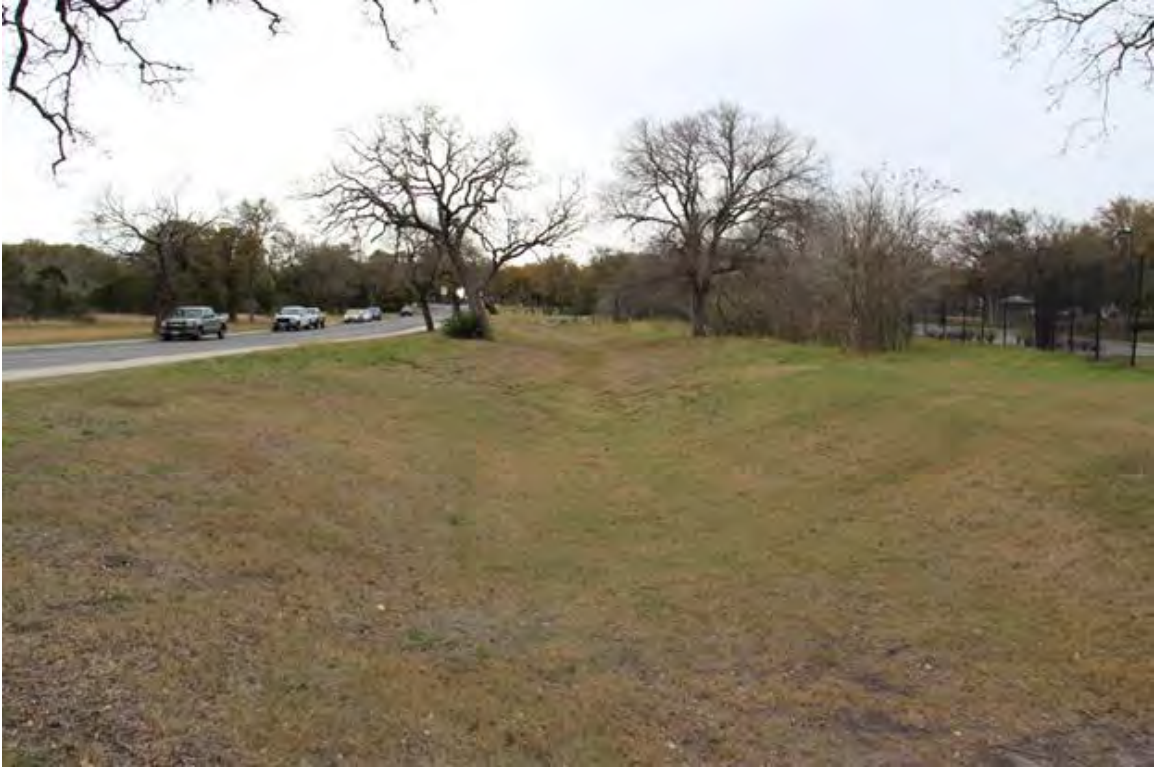
Figure 3-30. Roadside vegetated swale, San Antonio, Texas. Source: Tetra Tech
