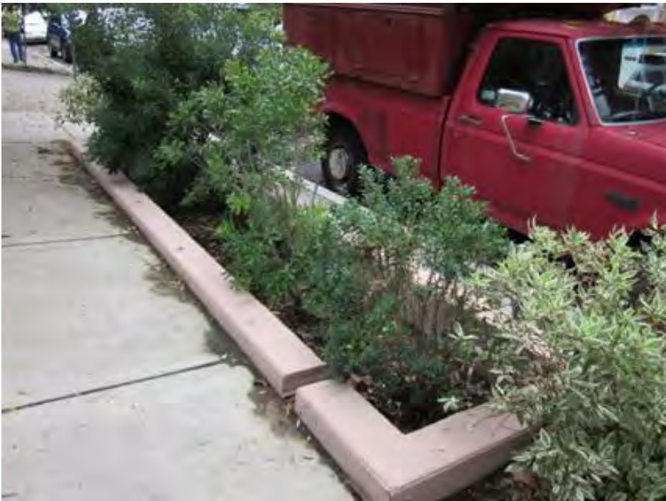
Figure 3-14. Planter box in an ultra-urban setting, Philadelphia, Pennsylvania. Source: Tetra Tech
