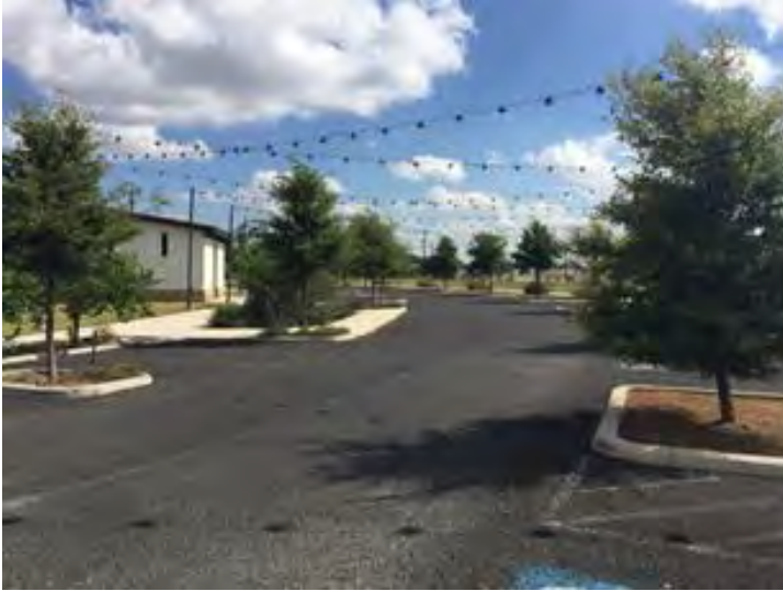
Figure 3-9. Porous asphalt parking lot, Mission Library, San Antonio Texas.
