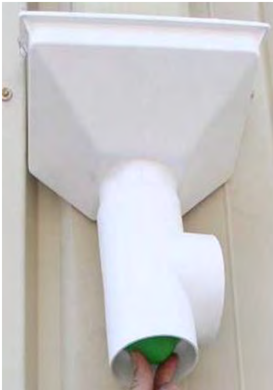
Figure B-9-14. Valve for a first-flush diverter. Source: North Carolina State University Department of Biological and Agricultural Engineering
