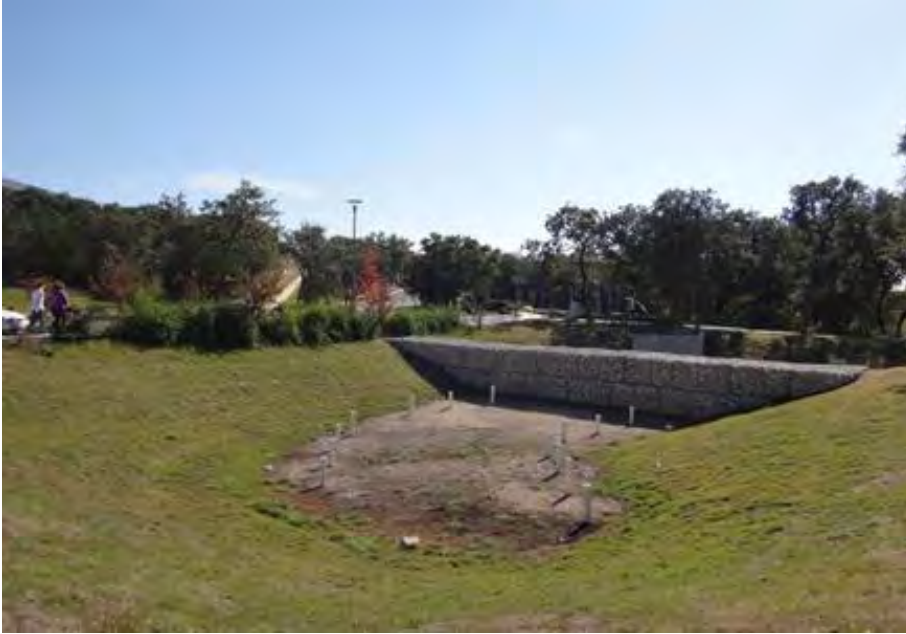
Figure3-17. Surface sand filter, Parman Library, San Antonio, Texas. Source: Bender Wells Clark Design
