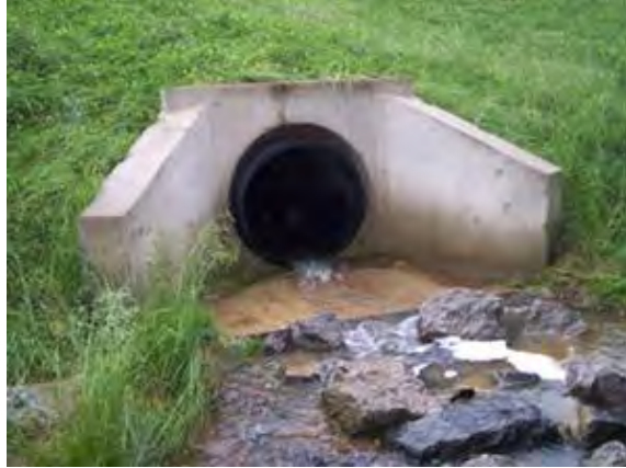
Figure B-8-10. Outfall. Source: Cranberry Township, Pennsylvania
