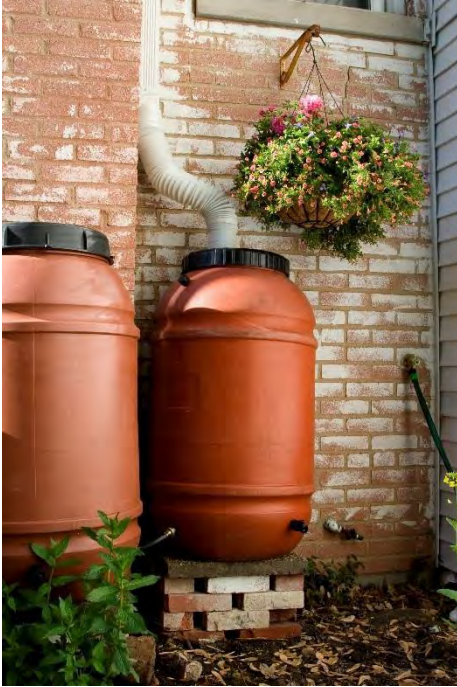
Figure 3-25. Residential rain barrel.
