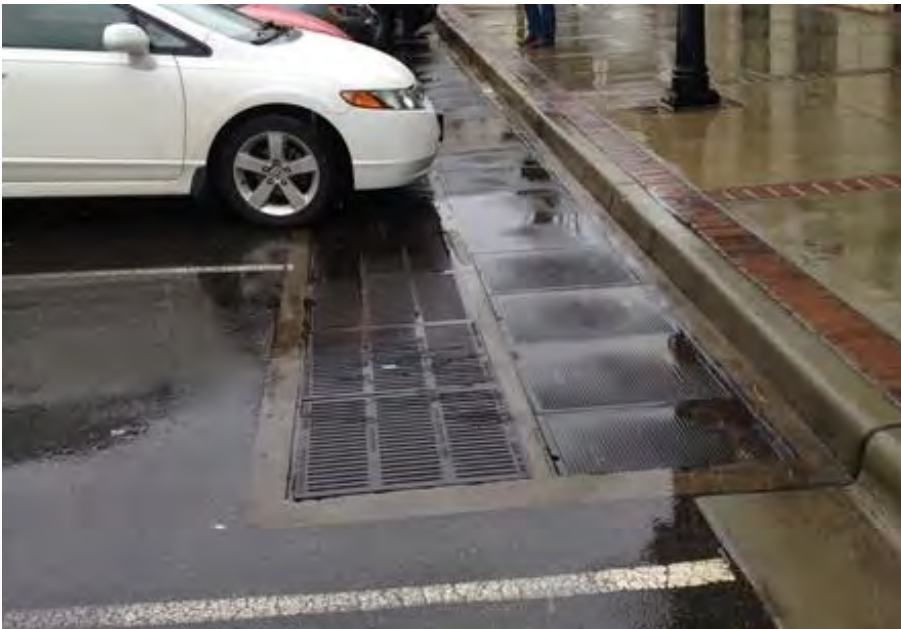
Figure 3-18. Subsurface sand filter, Raleigh, North Carolina. Source: Tetra Tech
