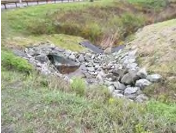
Figure B-8-9. Emergency spillway. Source: Randy Rath, the Huletts Current
