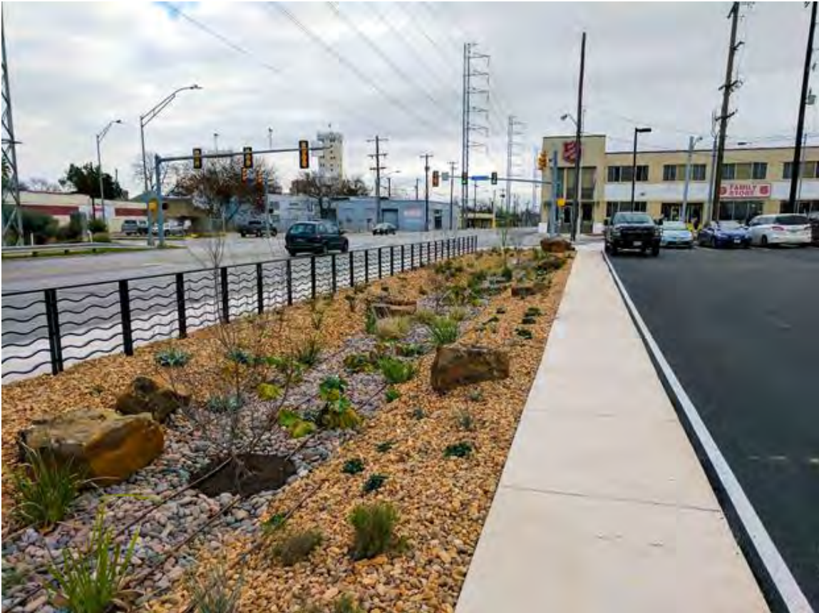
Figure 3-8. Bioswale that receives stormwater runoff from a parking lot, City of San Antonio Development Services Department, San Antonio, Texas.
