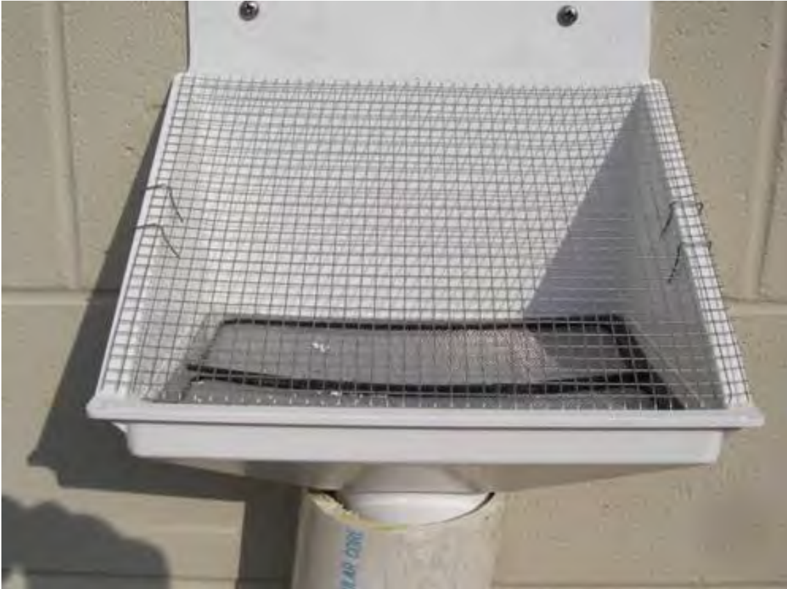
Figure B-9-12. Flow-through inlet filter. Source: Tetra Tech
