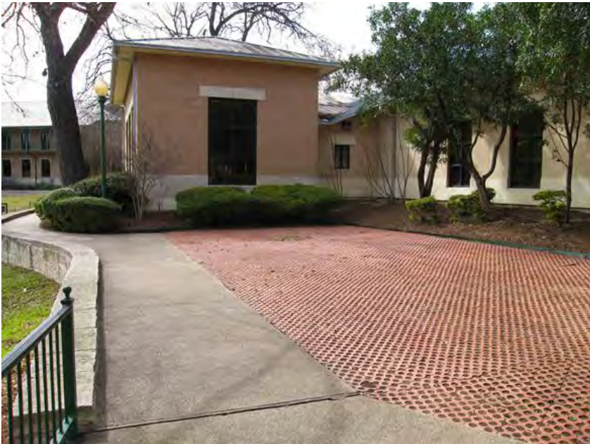
Figure 3-12. Concrete grid pavers used in an emergency vehicle access lane, San Antonio River Authority Main Office, San Antonio, Texas.
