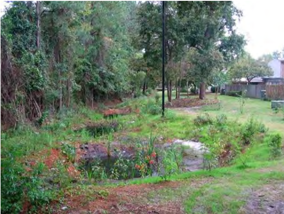
Figure 3-20. Small stormwater wetlands along the perimeter of a neighborhood, Wilmington, North Carolina. Source: Tetra Tech
