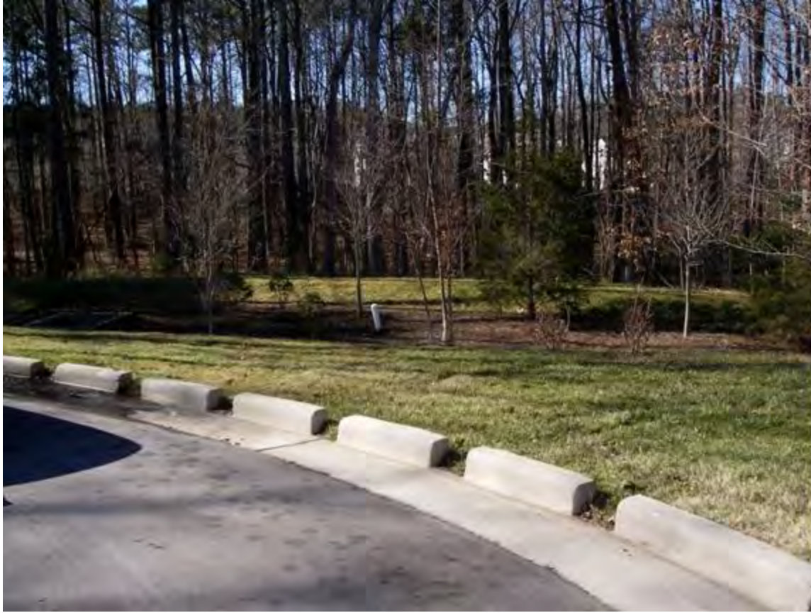
Figure B-13-4. Curb cuts and vegetated filter strip for a roadside bioretention area, Apex, North Carolina. Source: Tetra Tech
