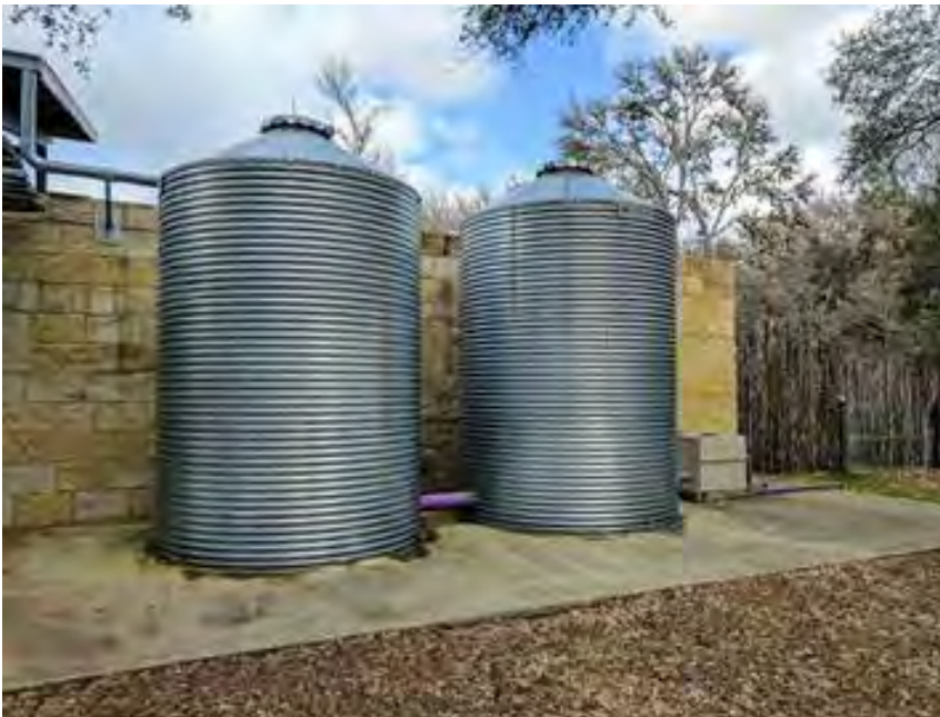
Figure B-9-3. Cistern greater than 2,000 psi on a concrete foundation, Phil Hardberger Park, San Antonio, Texas.
