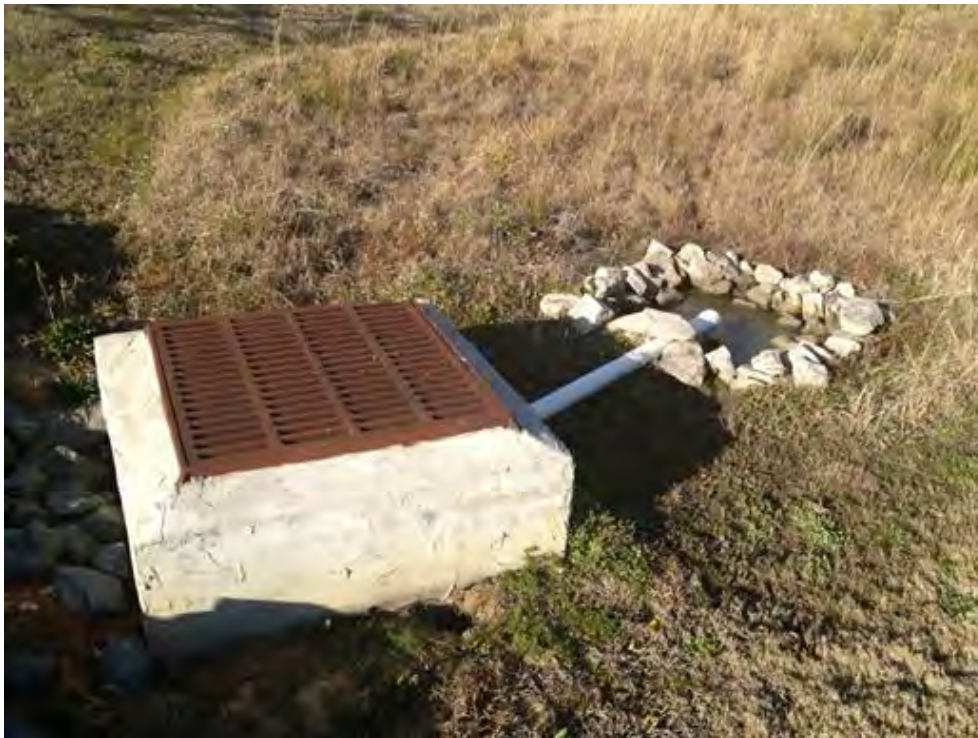
Figure B-7-7. A downturned inlet pipe with an orifice extends into a deep pool in a small stormwater wetland, Raleigh, North Carolina. Source: Tetra Tech
