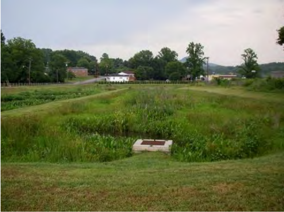
Figure 3-19. Large linear stormwater wetland, Lenoir, North Carolina. Source: Tetra Tech
