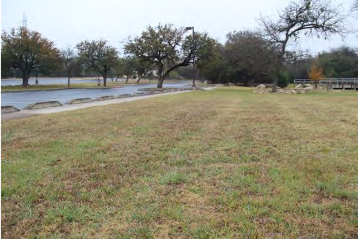
Vegetated Filter Strip at Oak Hills Church, San Antonio, Texas. Source: Tetra Tech
