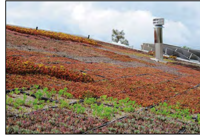
A modular extensive green roof in Fallbrook, California, was installed on the roof of a public library. Prefabricated plastic trays were planted with colorful varieties of stonecrop.
