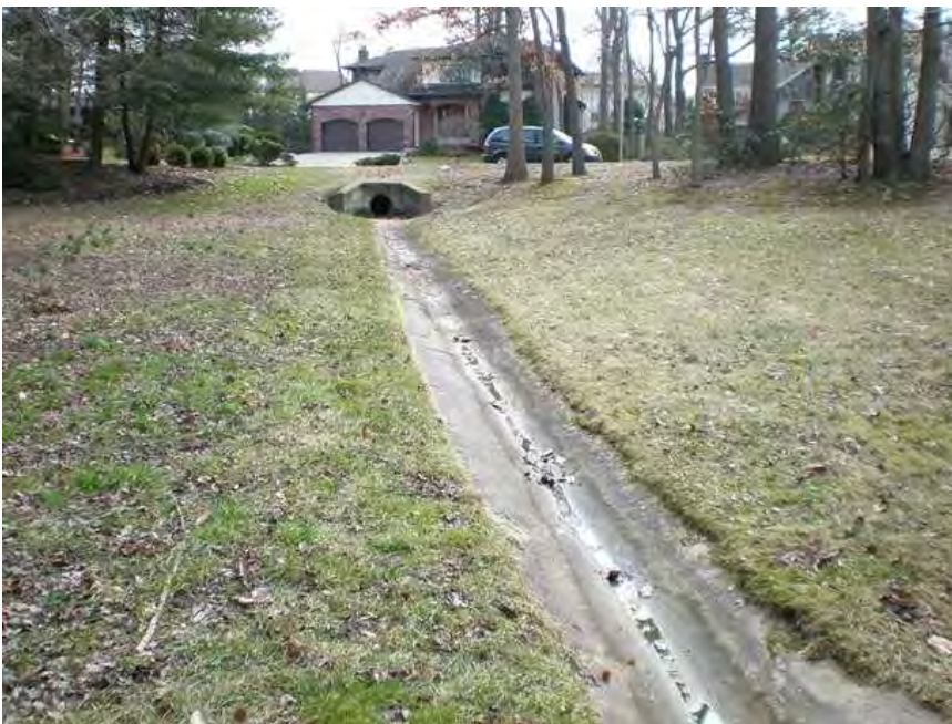
Figure B-8-3. Concrete trickle channel
