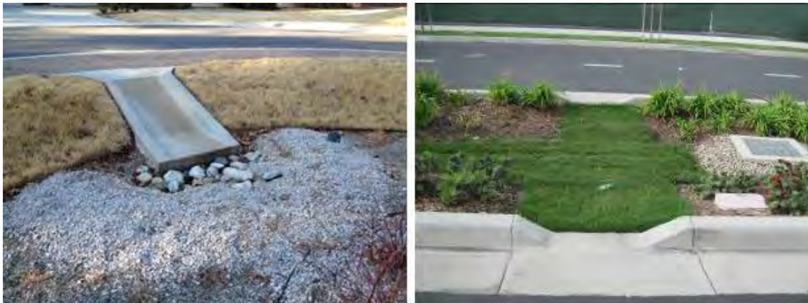
Figure B-13-5. Example curb cut configurations in Raleigh, North Carolina (left) and Downey, California (right). Source: Tetra Tech
