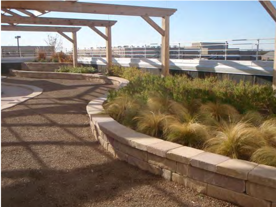
Figure 3-16. Intensive green roofs provide recreational, aesthetic, and educational opportunities in addition to stormwater benefits, James Madison High School Agriscience Building, San Antonio, Texas. Source: Bender Wells Clark Design
