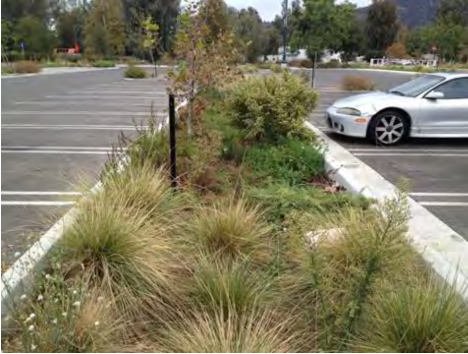
Figure 3-3. Parking lot bioretention area, Los Angeles, California. Source: Tetra Tech
