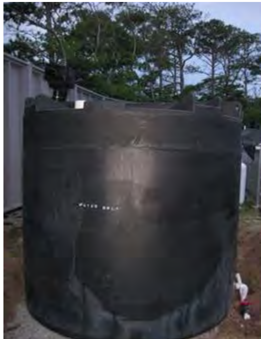
Figure 3-21. Typical plastic cistern, Pine Knoll Shores, North Carolina. Source Tetra Tech
