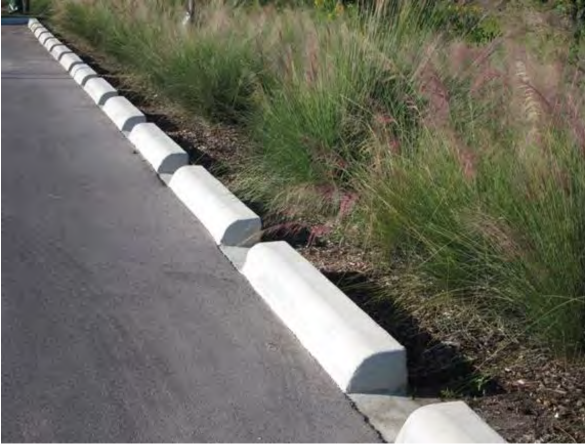
Figure B-13-3. Multiple, small curb cuts distribute parking lot runoff to bioretention area without erosive force at Mission Library, San Antonio, Texas. Source: Bender Wells Clark Design
