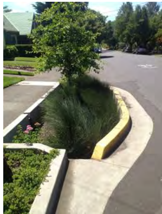
Figure 1-6. Bioretention curb pop-out, Portland, Oregon. Source: Tetra Tech
