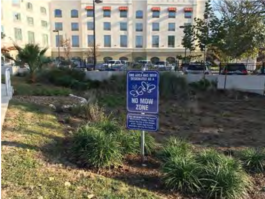
Figure B-1-14. Signage posted in front of ultra-urban bioretention area raises public awareness
