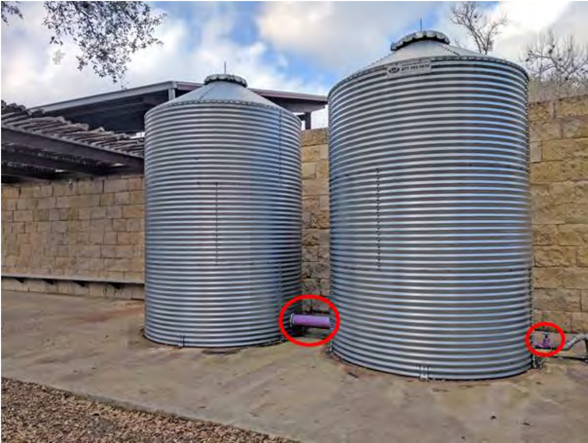
Figure B-9-19. Two cisterns with purple pipe connection at Phil Hardberger Park, San Antonio, Texas.
