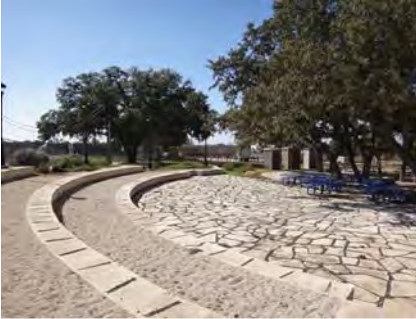
Figure 3-11. Permeable pavement pedestrian plaza, James Madison High School Agriscience Building, San Antonio, Texas. Source: Bender Wells Clark Design
