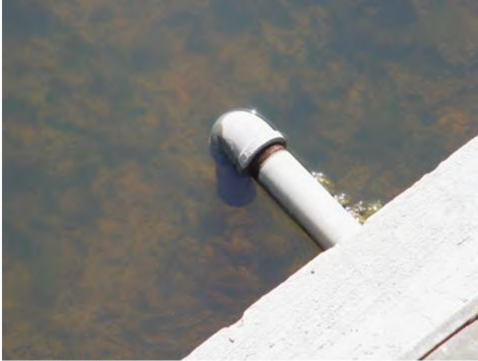
Figure B-13-15. Drawdown pipe with a downturned elbow
