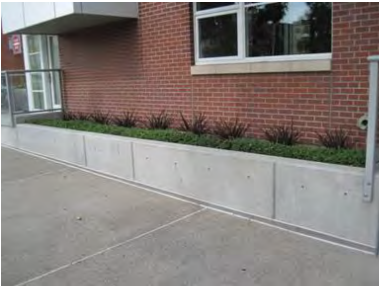
Figure B-4-1. Planter box inlet configuration, San Diego, California. Source: Tetra Tech
