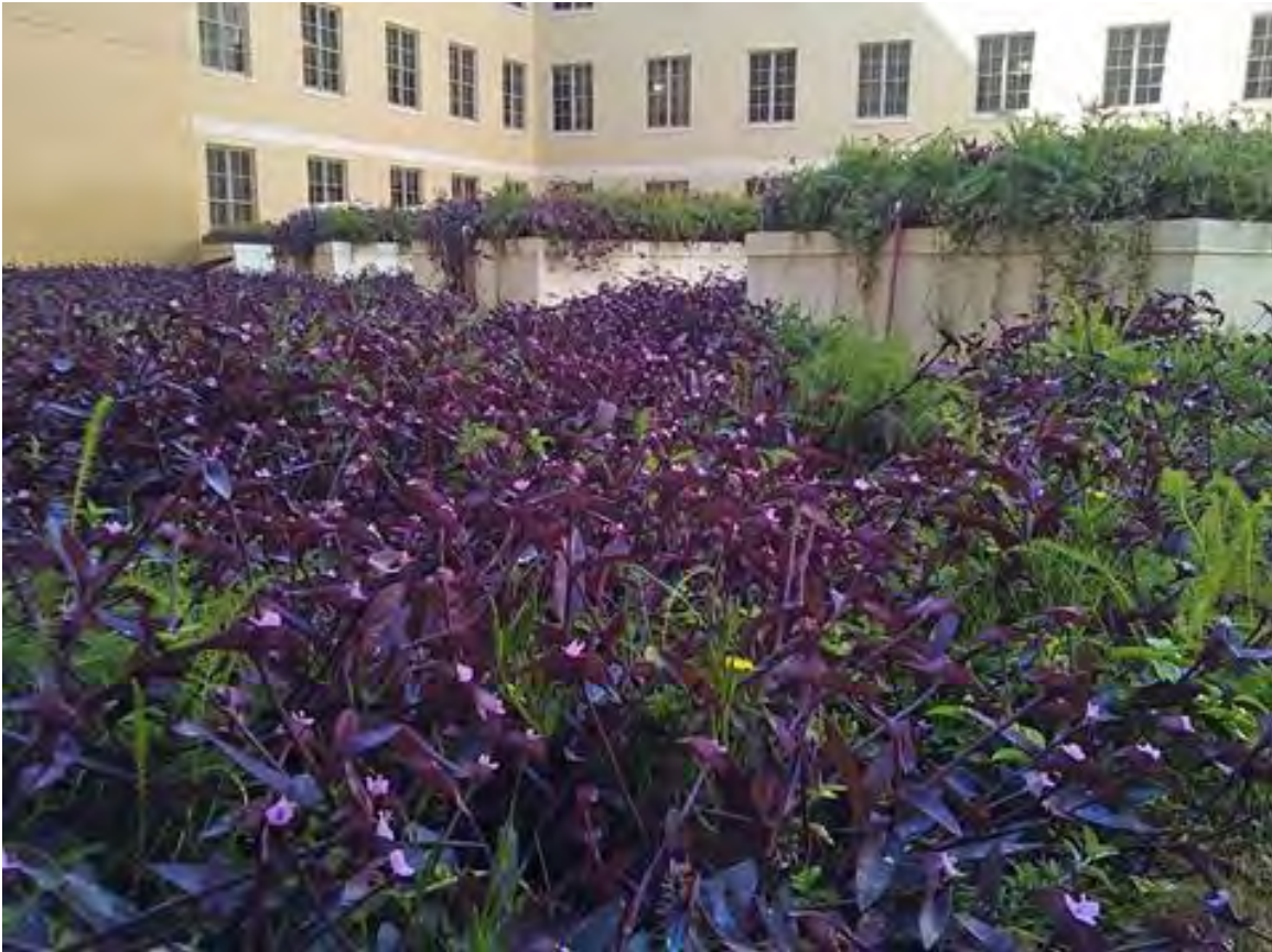
Figure 3-15. Extensive green roofs reduce stormwater runoff while providing cooling effects, Hipolito F. Garcia Federal Building and United States Courthouse, San Antonio, Texas. Source: Joss Growers
