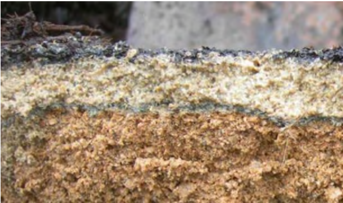
Figure 4-2. Accumulated fines layer as a result of improper construction sequencing. Source: North Carolina State University Department of Biological and Agricultural Engineering
