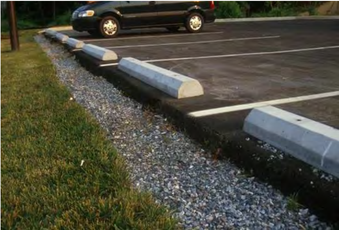
Figure B-1-5. Gravel fringe and vegetated filter strip pretreatment, Louisburg, North Carolina. Source: North Carolina State University Department of Biological and Agricultural Engineering
