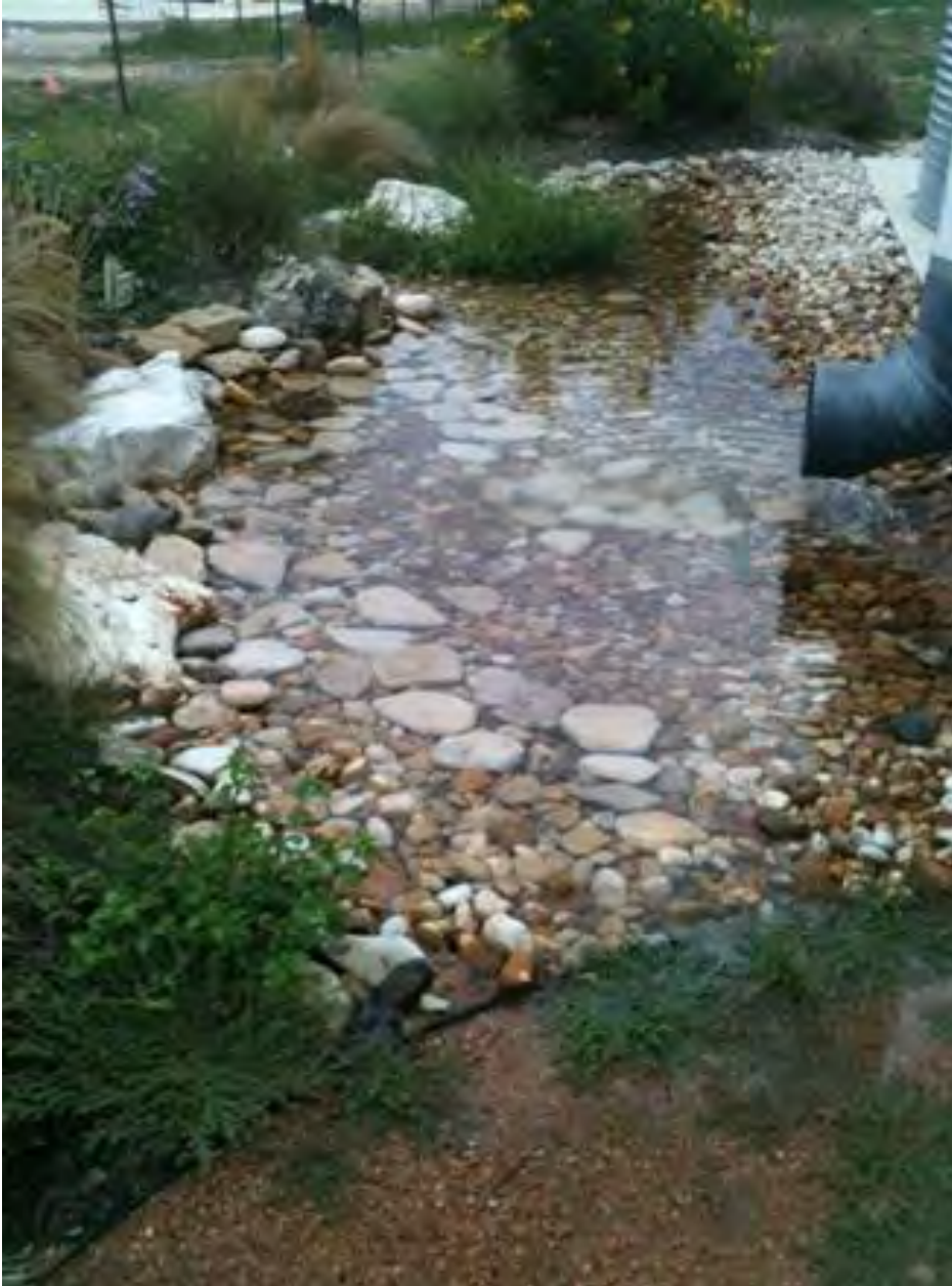
Figure B-1-16. Overflow from a rainwater cistern is discharged to a cobbled bioretention area at Mission Library, San Antonio, Texas. Source: Bender Wells Clark Design
