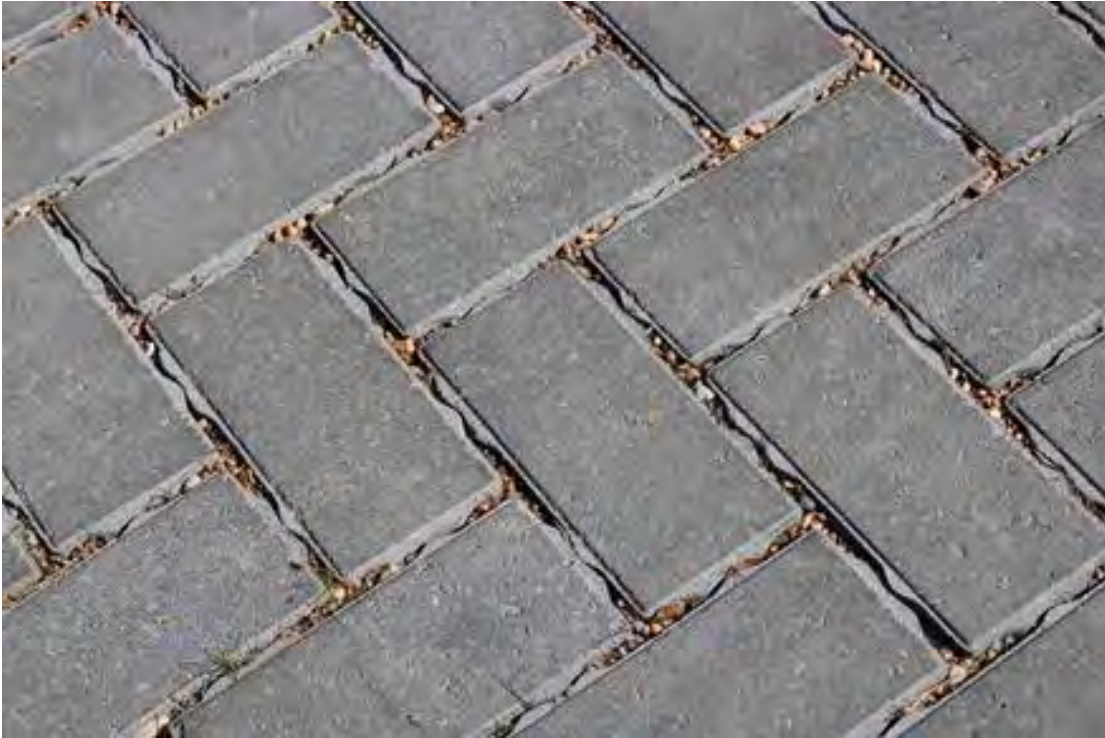
Figure B-3-7. Example of Permeable Interlocking Concrete Pavers (PICP) in a herringbone pattern at San Antonio River Authority Main Office, San Antonio, Texas.
