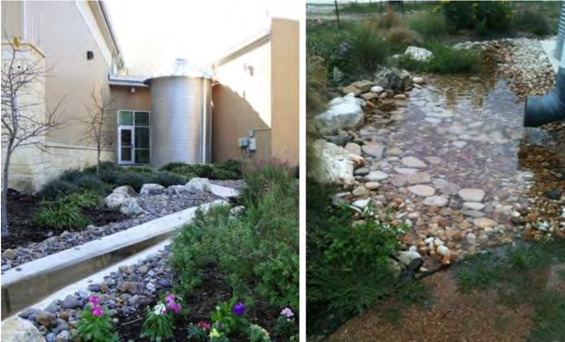
Figure B-9-18. A concrete channel (left) directs overflow away from the building at the Shavano Park Fire Station, Shavano Park, Texas; and a cistern overflows to an adjacent bioretention area lined with cobble (right) at Mission Library, San Antonio, Texas. Source: Bender Wells Clark Design
