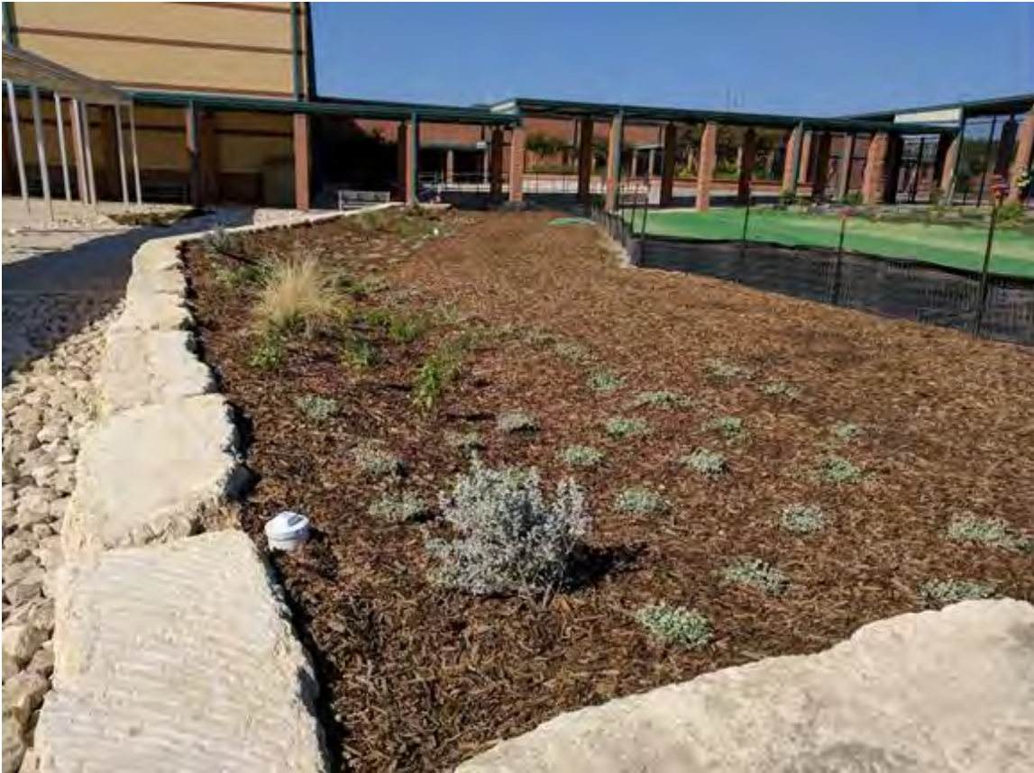
Figure 3-7. Bioretention in a common area, Hector Garcia Middle School, San Antonio, Texas.
