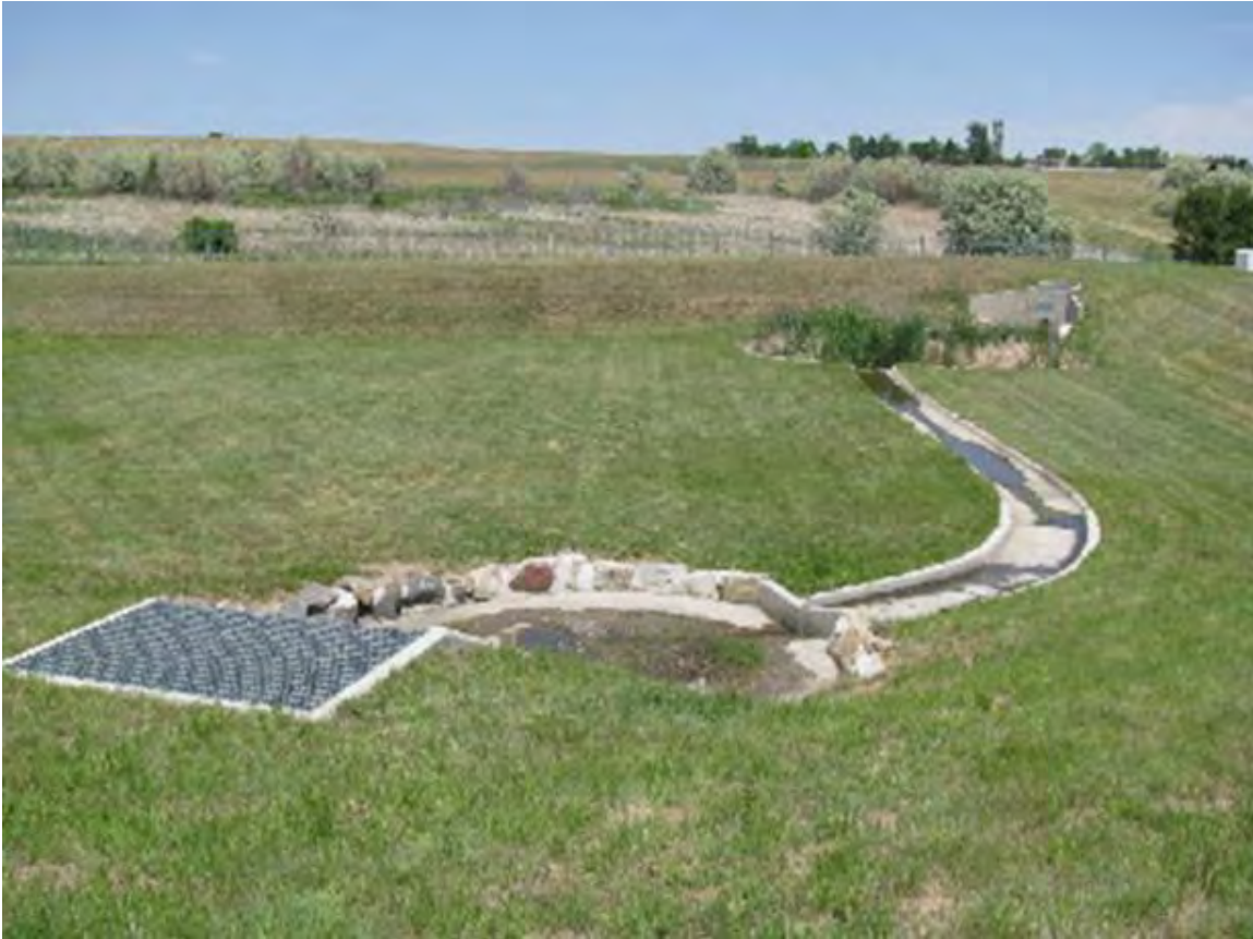
Extended Detention Basin in Grant Ranch, Colorado. Source: Urban Drainage Flood Control District
