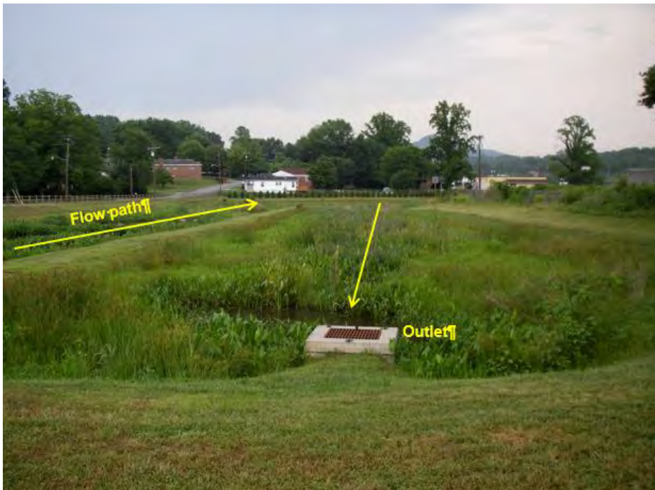
Figure B-7-4. An earthen berm elongates the flow path in a racetrack-style stormwater wetland where the inlet and outlet are located in close proximity, Lenoir, North Carolina. Source: Tetra Tech
