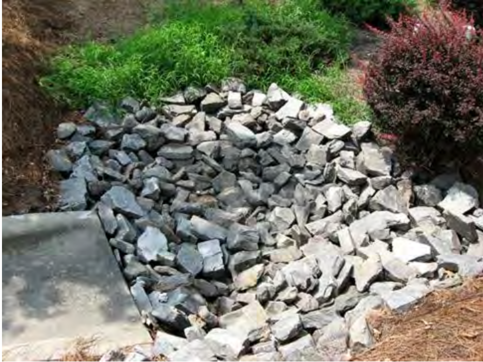
Figure B-13-7. Angular stone flow dissipater/forebay, Cary, North Carolina. Source: Tetra Tech
