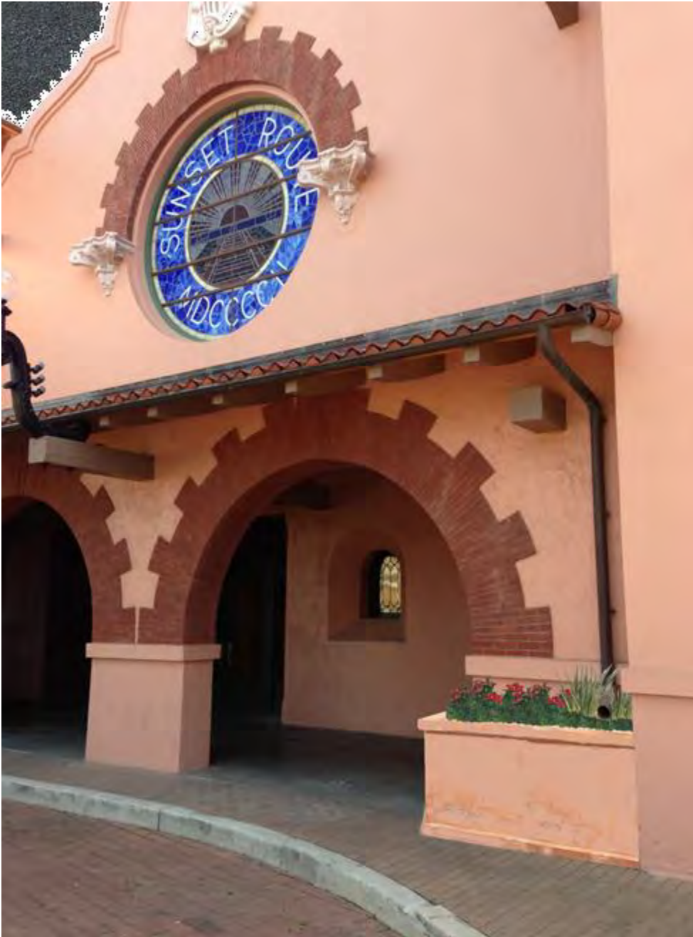
Rendering of example planter box retrofit to treat rooftop runoff at Sunset Station. San Antonio, Texas.
