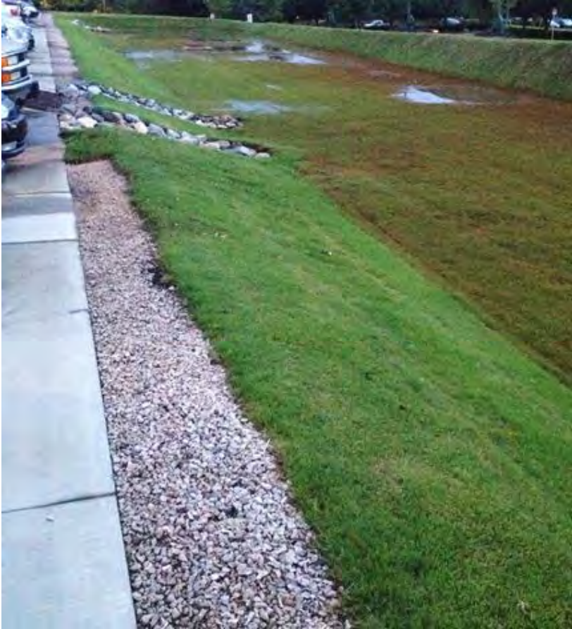
Figure 3-32. Vegetated filter strip surrounding a bioretention area in a parking lot, Raleigh, North Carolina. Source: Tetra Tech
