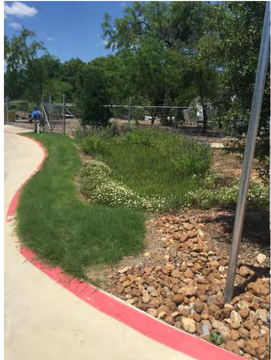
Figure 1-5. Bioretention cell adjacent to roadway, Mission Reach Operations Center, San Antonio, Texas.
