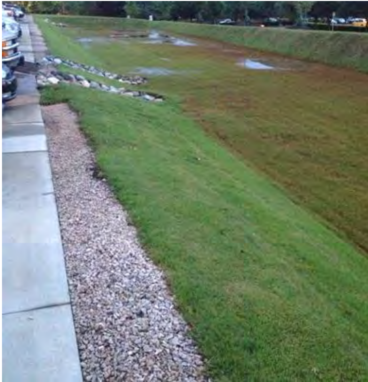
Figure 3-1. Treatment train featuring a vegetated filter strip pretreating stormwater runoff before entering a grassed bioretention area, Raleigh, North Carolina. Source: Tetra Tech
