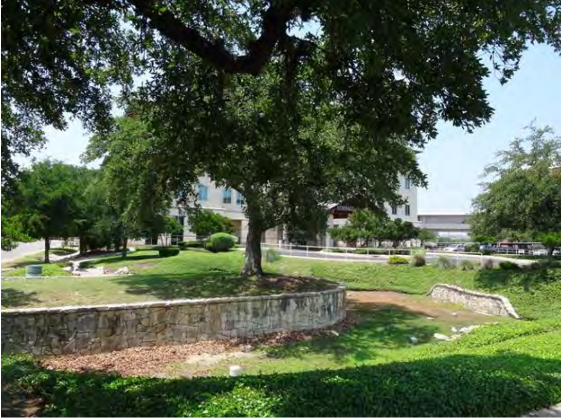
Surface sand filter at Remington Oaks, San Antonio, Texas. Source: Bender Wells Clark Design
