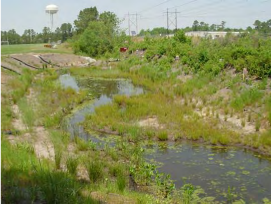
Figure B-7-3. A sinuous pattern increases the flow path in a stormwater wetland, Wilmington, North Carolina. Source: Tetra Tech
