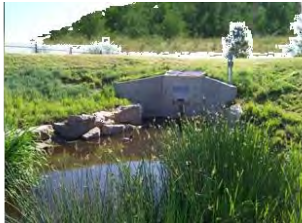
Figure B-8-8. Vertical trash rack with flared wing walls. Source: Urban Drainage Flood Control District
