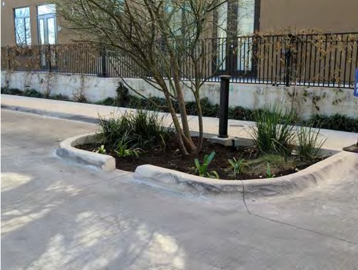
Figure 3-6. Rain garden pop-out incorporated with on-street parking, River House, San Antonio, Texas.
