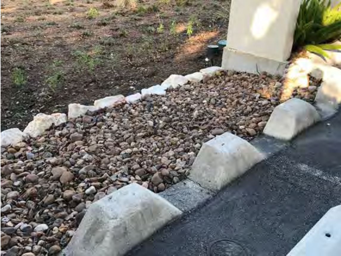
Figure B-13-2. A typical curb cut, San Antonio, Texas.
