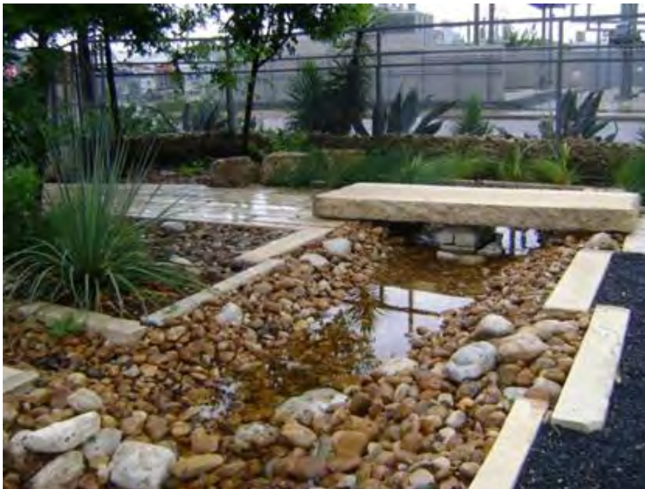
Figure B-1-15. Cobbled bioretention area that invites pedestrian interaction at the offices of Bender Wells Clark Design. Source: Bender Wells Clark Design
