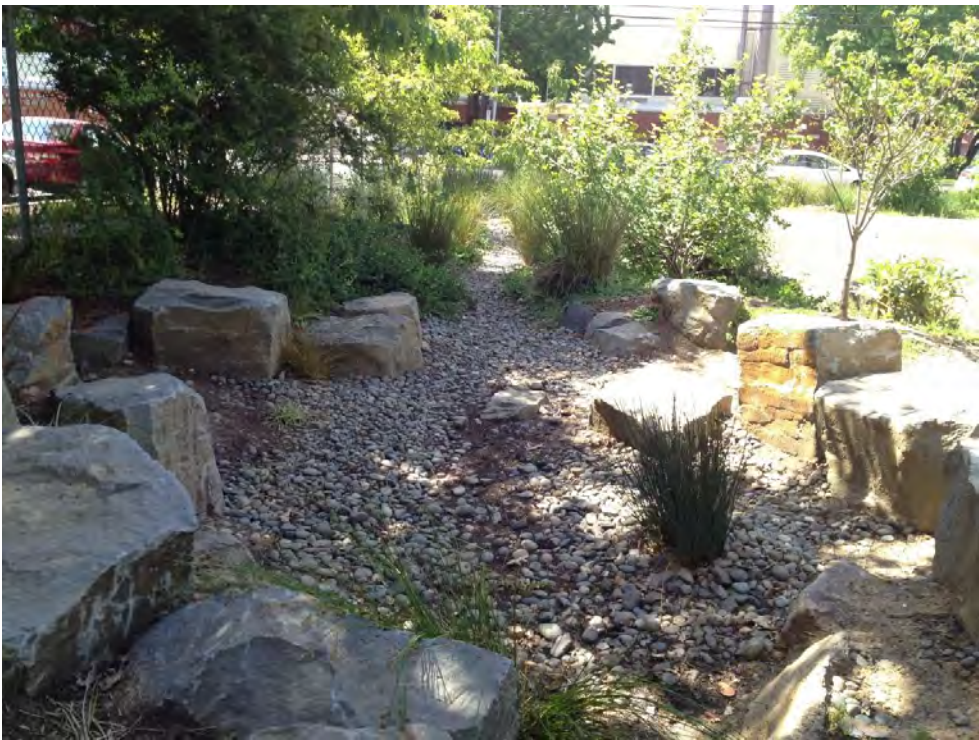
Figure 1-4. A bioretention area provides attractive landscaping that is also functional, Portland, Oregon. Source: Tetra Tech
