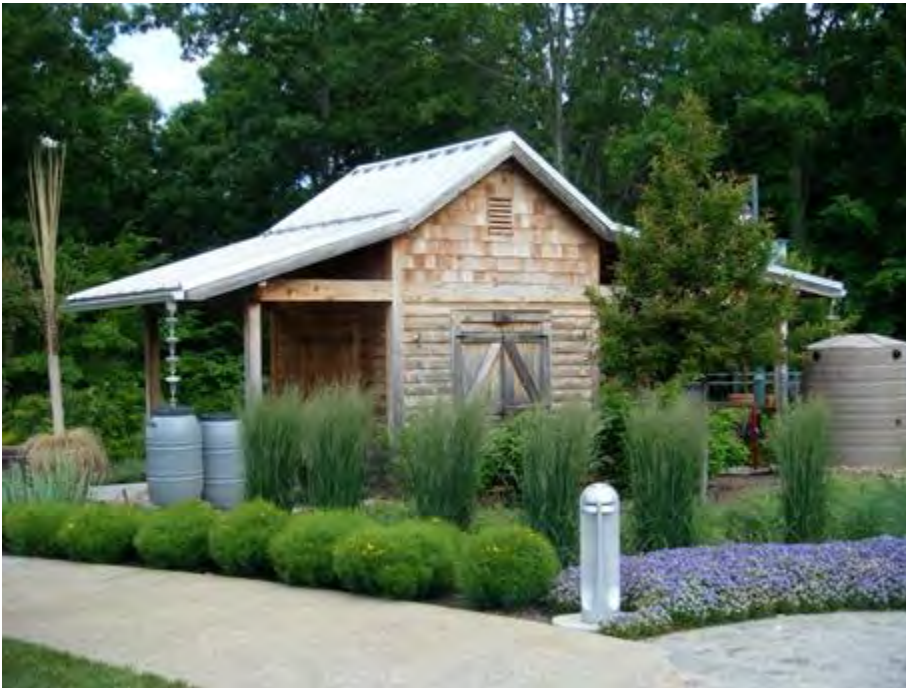
Figure 3-26. Rain barrels adequately sized for contributing roof area, Asheville, North Carolina. Source: Tetra Tech
