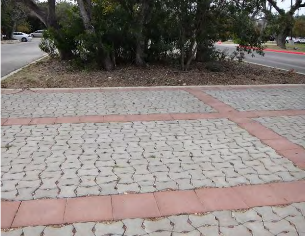
Permeable pavement parking stalls at the Oaks at University Business Park, San Antonio, Texas. Source: Bender Wells Clark Design
