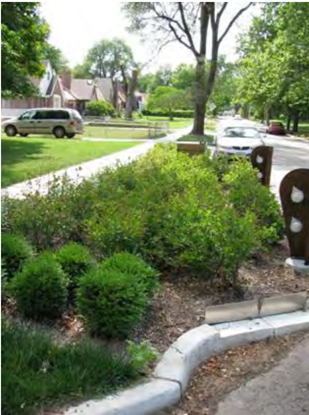
Figure 4-17. Outlet of a roadside bioretention pop-out equipped with a V-notch weir for flow monitoring. Source: Tetra Tech
