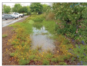
DESCRIPTION: A rain garden is a form of bioretention designed to have aesthetic appeal as well as a stormwater function. Rain gardens are commonly a depressed landscaped basin where runoff from roofs or paving infiltrates into the soil.
