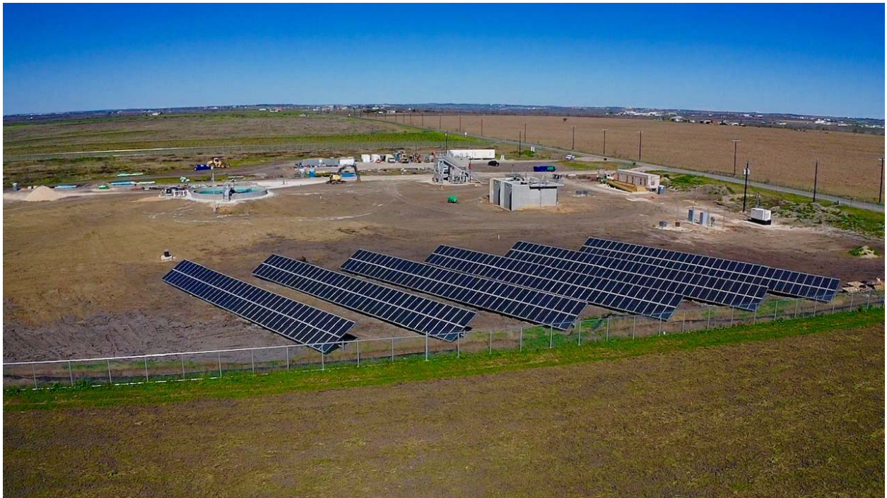
Martinez IV WWTP, Bexar County
