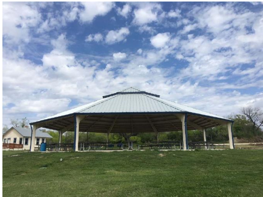
John William Helton San Antonio River Nature Park Pavilion Floresville, Wilson County
