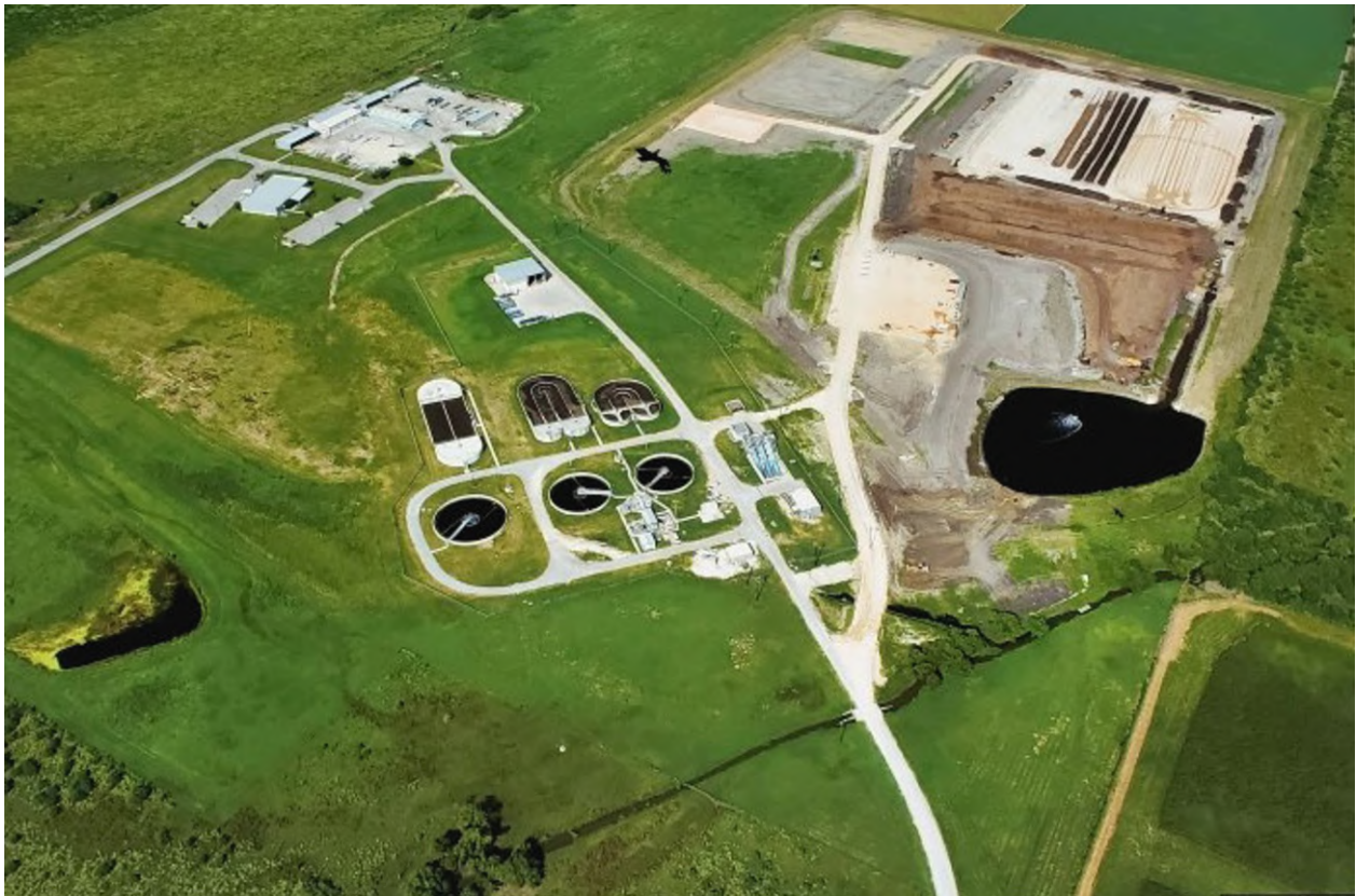
Martinez II Wastewater Treatment Plant and Recycling Facility Converse, Bexar County
