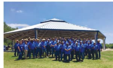
Watershed and Park Operations, John William Helton San Antonio River Nature Park Pavilion, Wilson County
