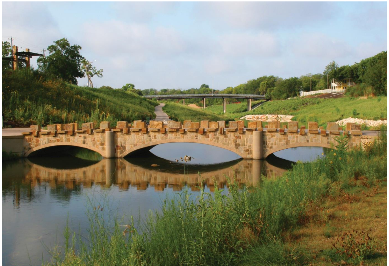
San Antonio River Improvement Project Mission Reach, Bexar County
