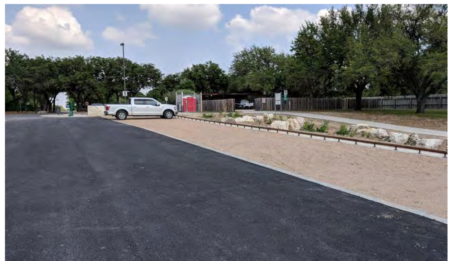
Figure 77: Leon Vista Trailhead – Permeable Parking
