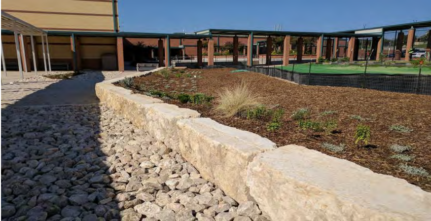
Figure 74: Hector Garcia Middle School – Bioretention Area
