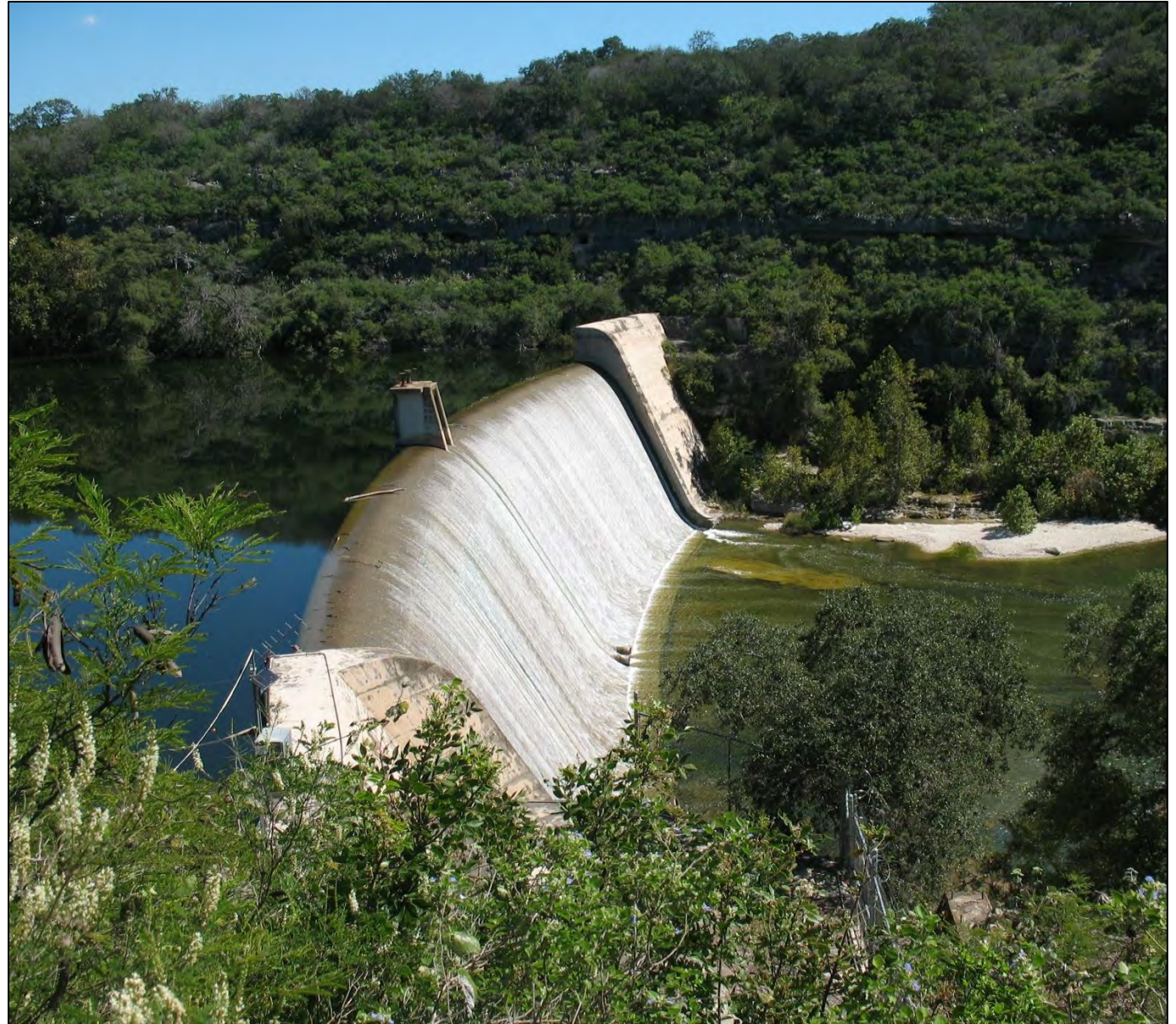
Figure 42: Medina Diversion Lake Dam, Medina River Watershed
