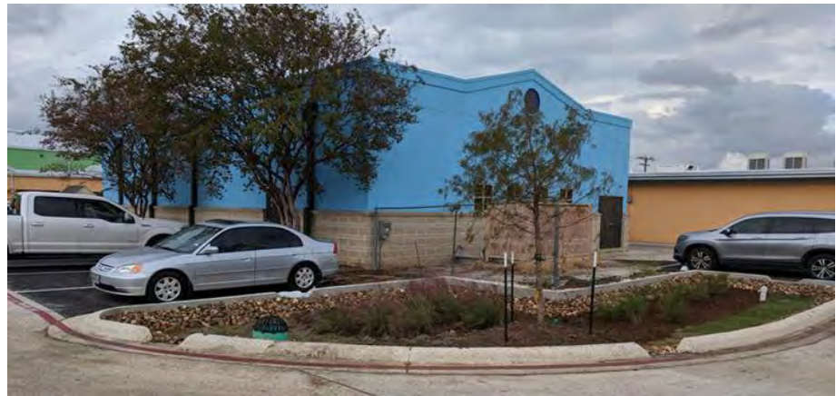
Figure 75: Neighborhood Place Community Center – Bioretention
