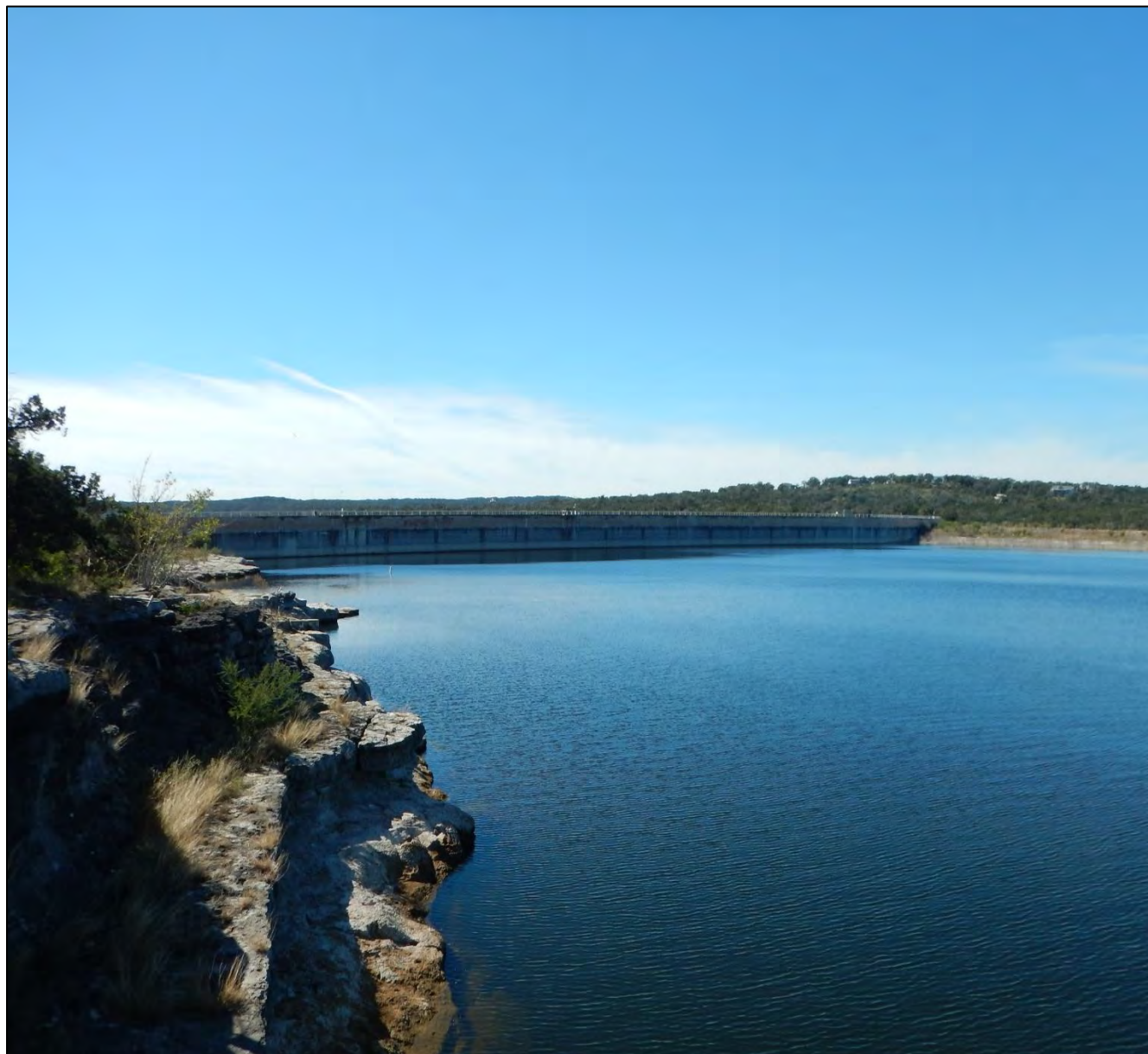
Figure 40: Medina Lake Dam, Medina River Watershed
