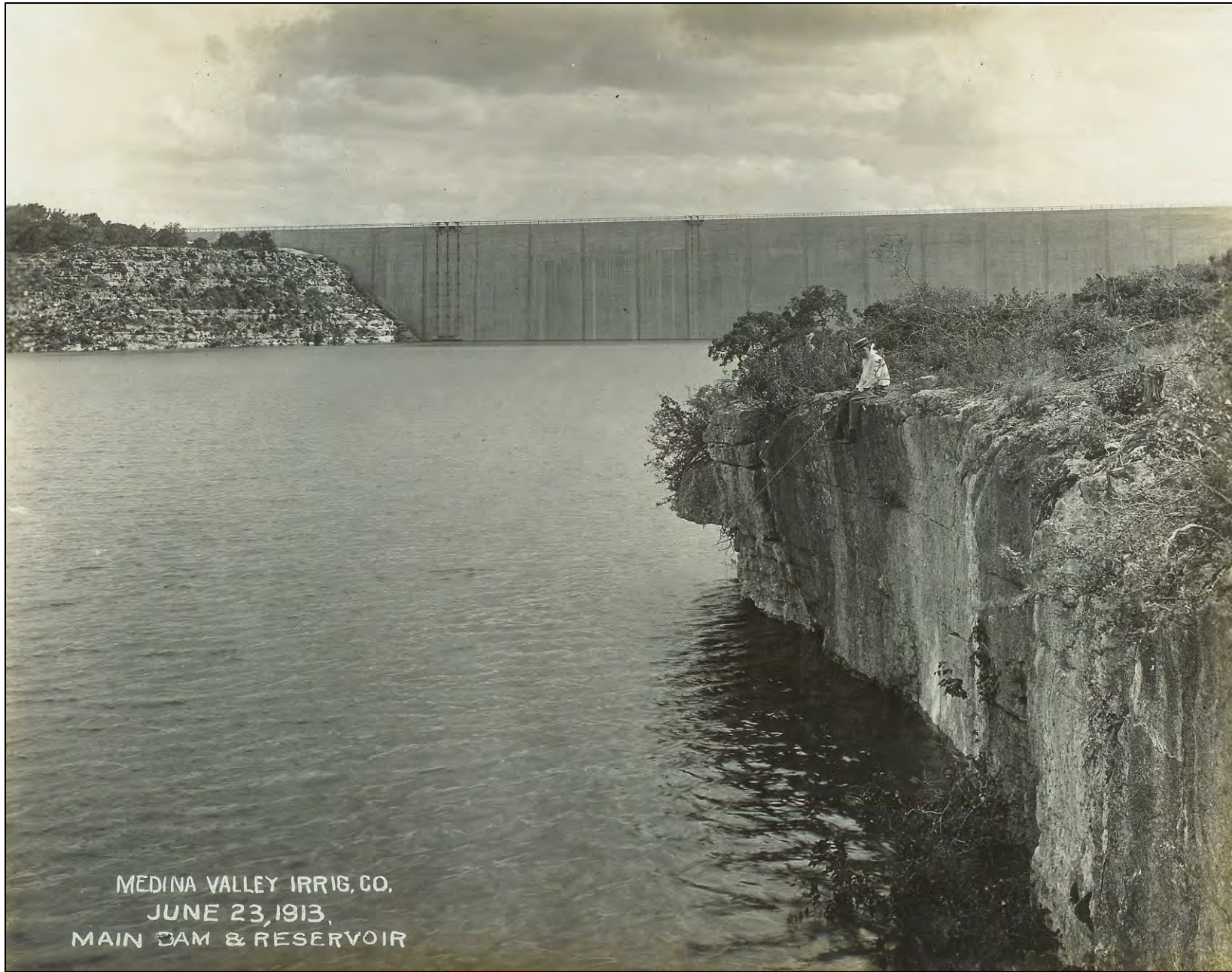
Figure 41: Medina Lake Dam, Medina Valley Irrigation Company, June 23, 1913
