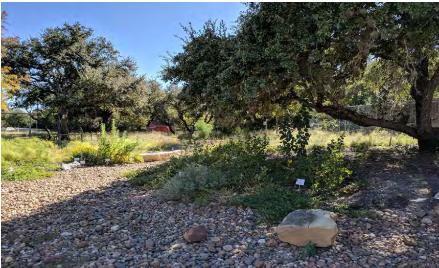
Figure 76: Rudder Middle School – Swale and Bioretention Areas
